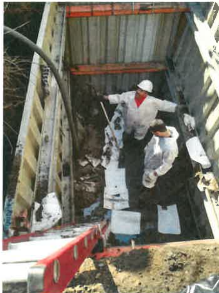
EXPOSED UST AFTER DEWATERING
