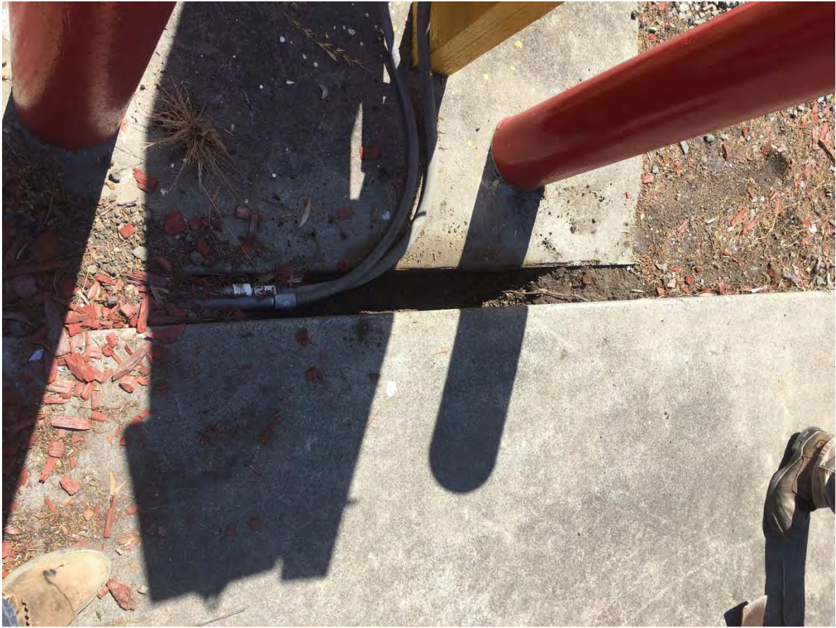
Excavation E-4 between concrete pads, note flexible electrical conduits in trench
