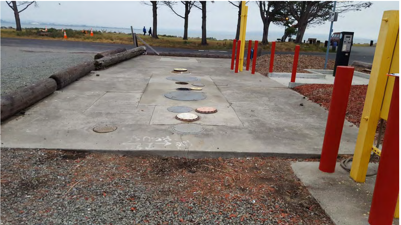
25,000-gal UST, looking west toward roadway, contaminated soil visible in left foreground (Area E-2)
