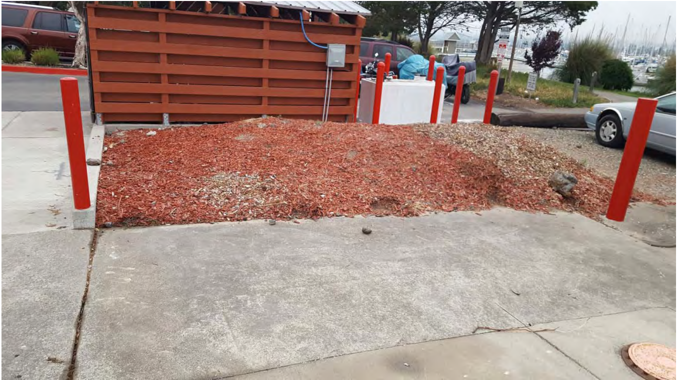
Stained soil at intersection of UST pad and sidewalk (Area E-3)
