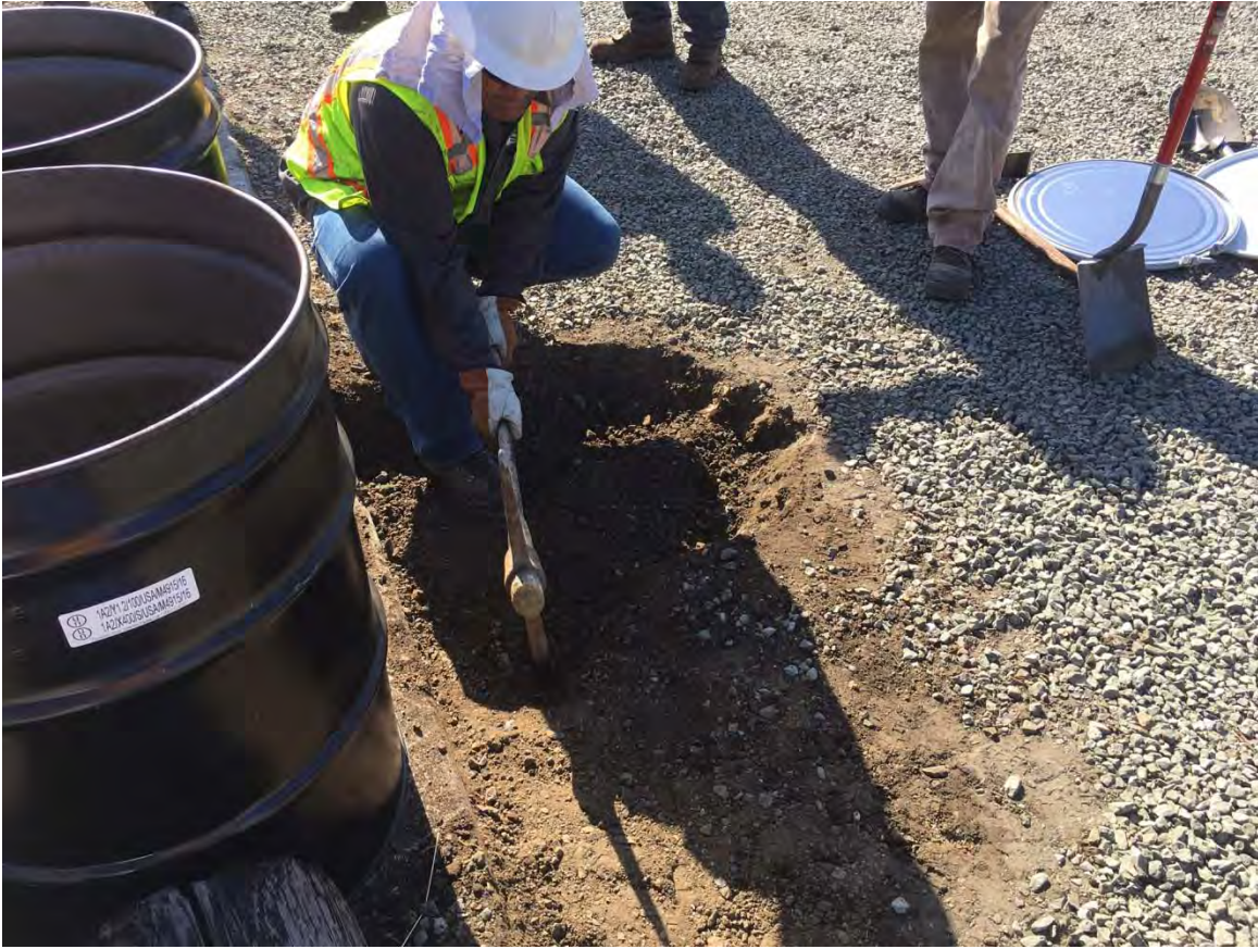
Excavating in Area E-1, south of UST
