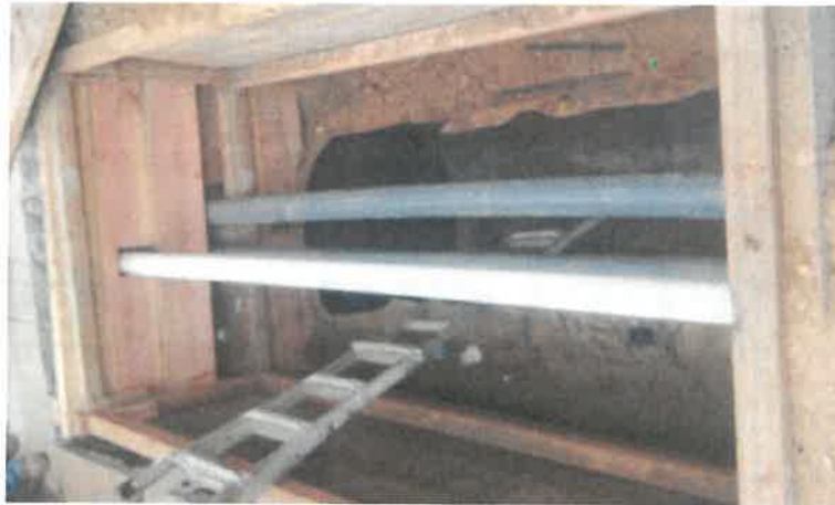
UST READY TO REMOVED FROM EXCAVATION
