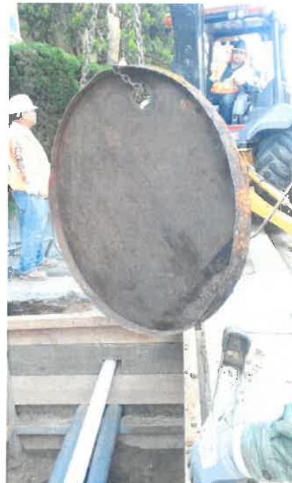
TANK REMOVAL IN PROCESS
