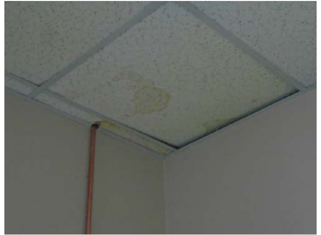
22. View of stained ceiling tile
