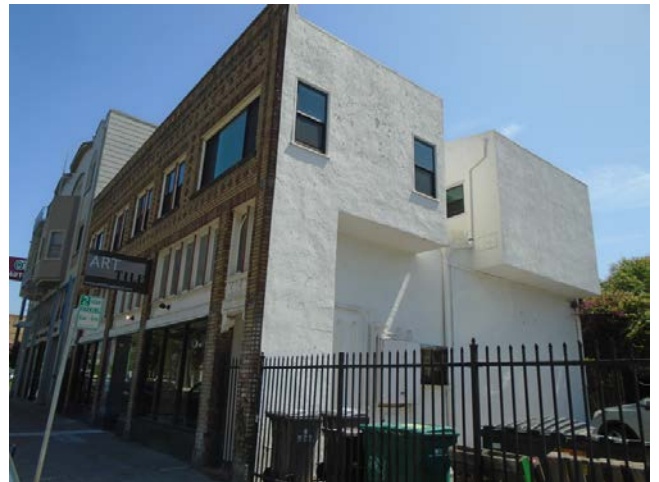
24. View of the northeast adjacent property (4336-4344 Broadway)
