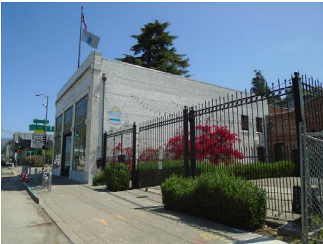
27. View of the south adjacent property
