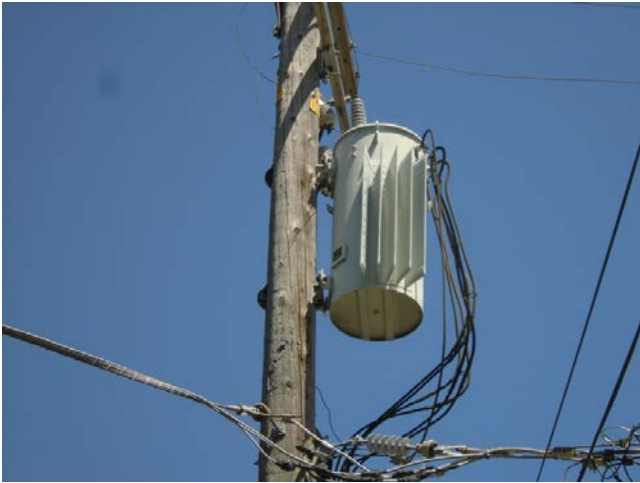
13. Pole-mounted transformer
