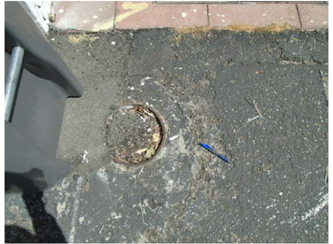
10. View of former sign post in the northern corner of the parking lot
