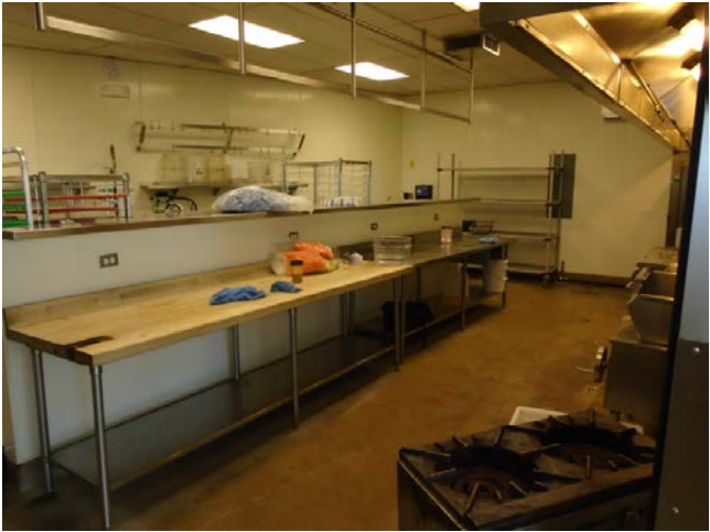
18. View of typical interior area
