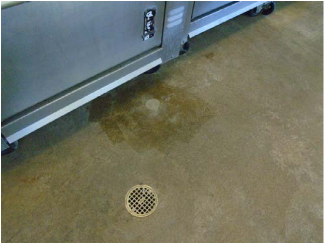
20. View of representative floor drain in kitchen and food prep areas
