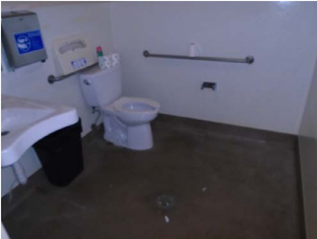
19. View of typical bathroom
