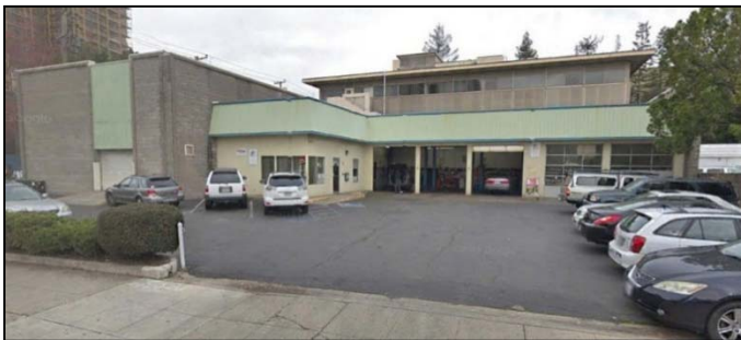
240 West MacArthur Boulevard
