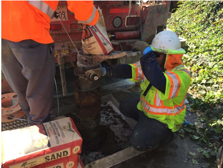
Drilling of EX-3
