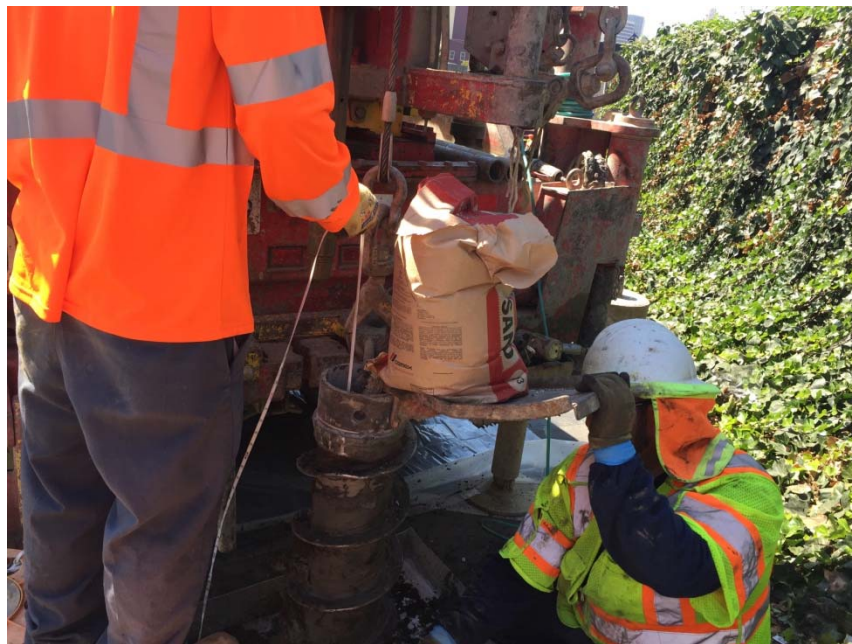
Construction of EX-3
