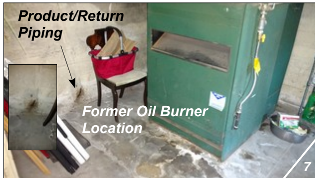
Photograph No. 6 – North view of interior of basement (northeast corner) showing residual staining at base of foundation stem wall; oil product reportedly issued through cracks of stem wall during period of heavy rain in December 2016 and cleaned up by property owner thereafter; basement floor approximately 4 to 4.5 feet below elevation of driveway at location of former UST (WGE, 8/9/17).
