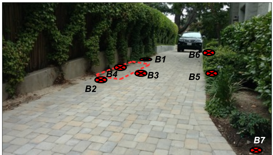
Photograph No. 2 – Southeast view of driveway along east side of residence, showing approximate location and lateral limits of former 300-gallon Heating Oil UST excavation (shown as red dashed line) and proposed investigation soil borings and field point IDs (WGE, 8/23/17).
