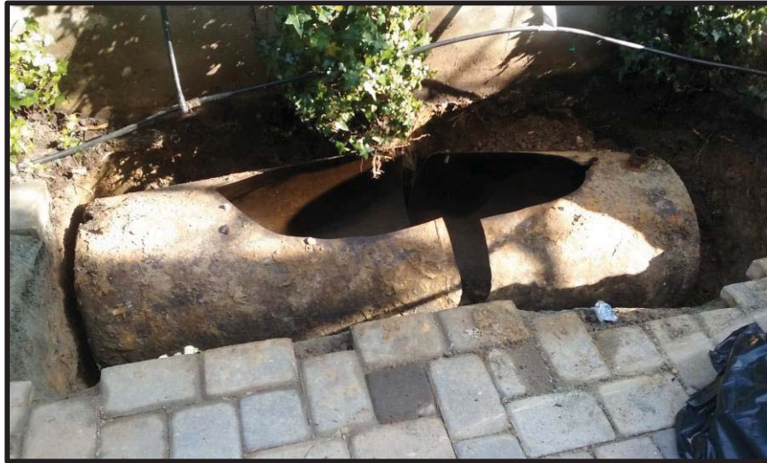
TANK IN EXCAVATION
