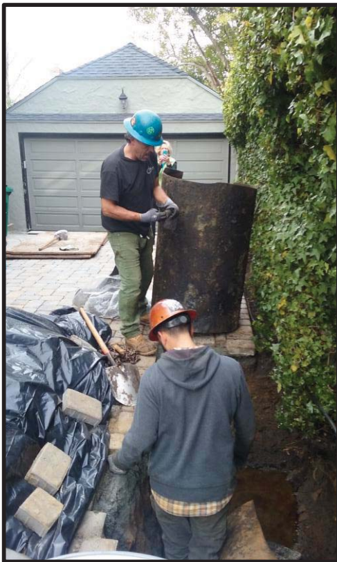
TANK REMOVAL IN PROGRESS
