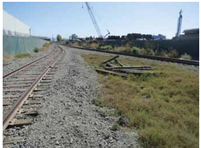
Picture 12 – Rail spur along southern portion of the subject Property
