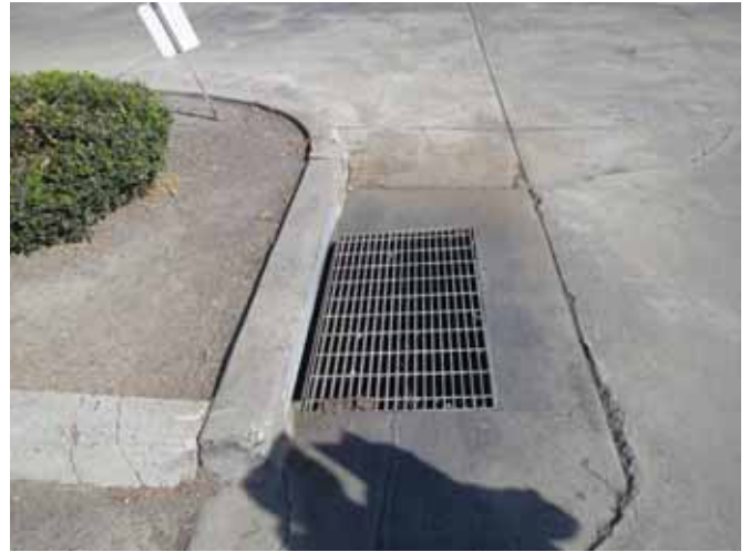
Picture 16 – Exterior surface drain
