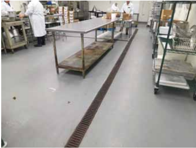
Picture 13 – Trench drain in food processing area
