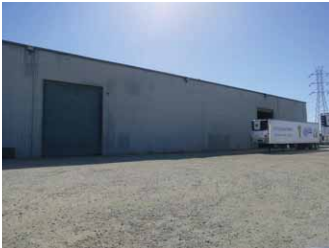
Picture 8 – Western adjoining property
