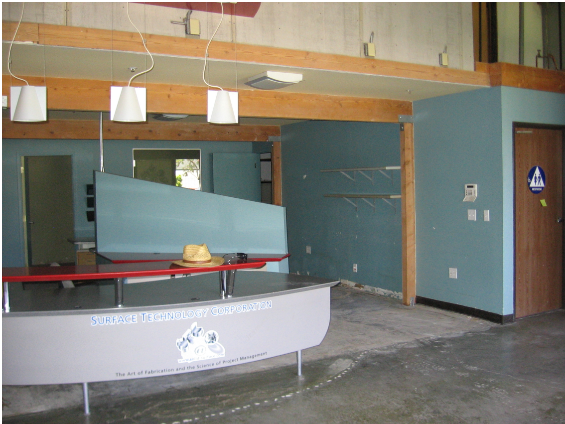
Photograph 4 - View of front office area inside building
