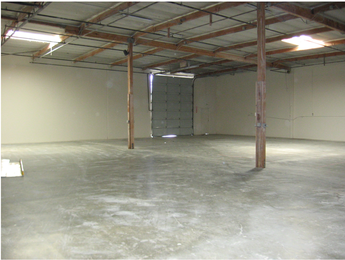
Photograph 5 - Part of warehouse area inside building
