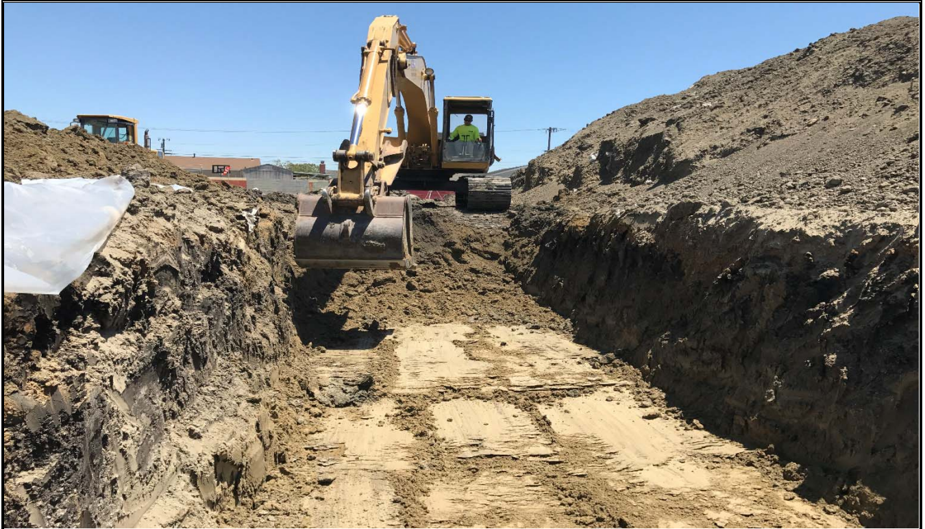
Photo 1. Excavation of PCE-impacted area (Batches 1 and 2).
