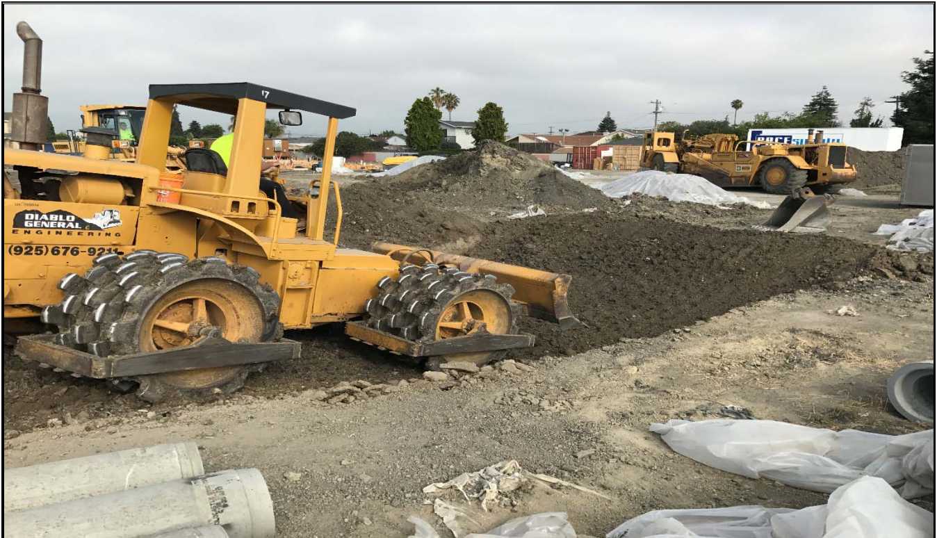
Photo 5. Backfilling and compaction of excavation.
