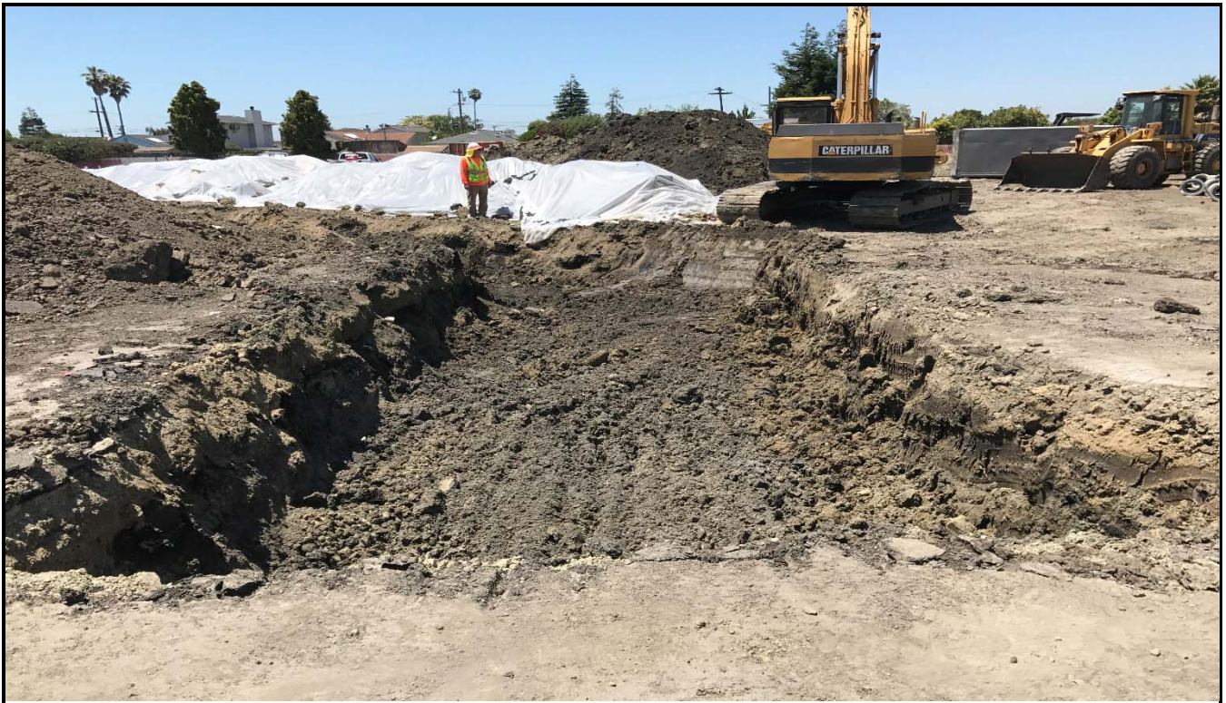
Photo 2. Excavation of PCE-impacted area (Batch 3).
