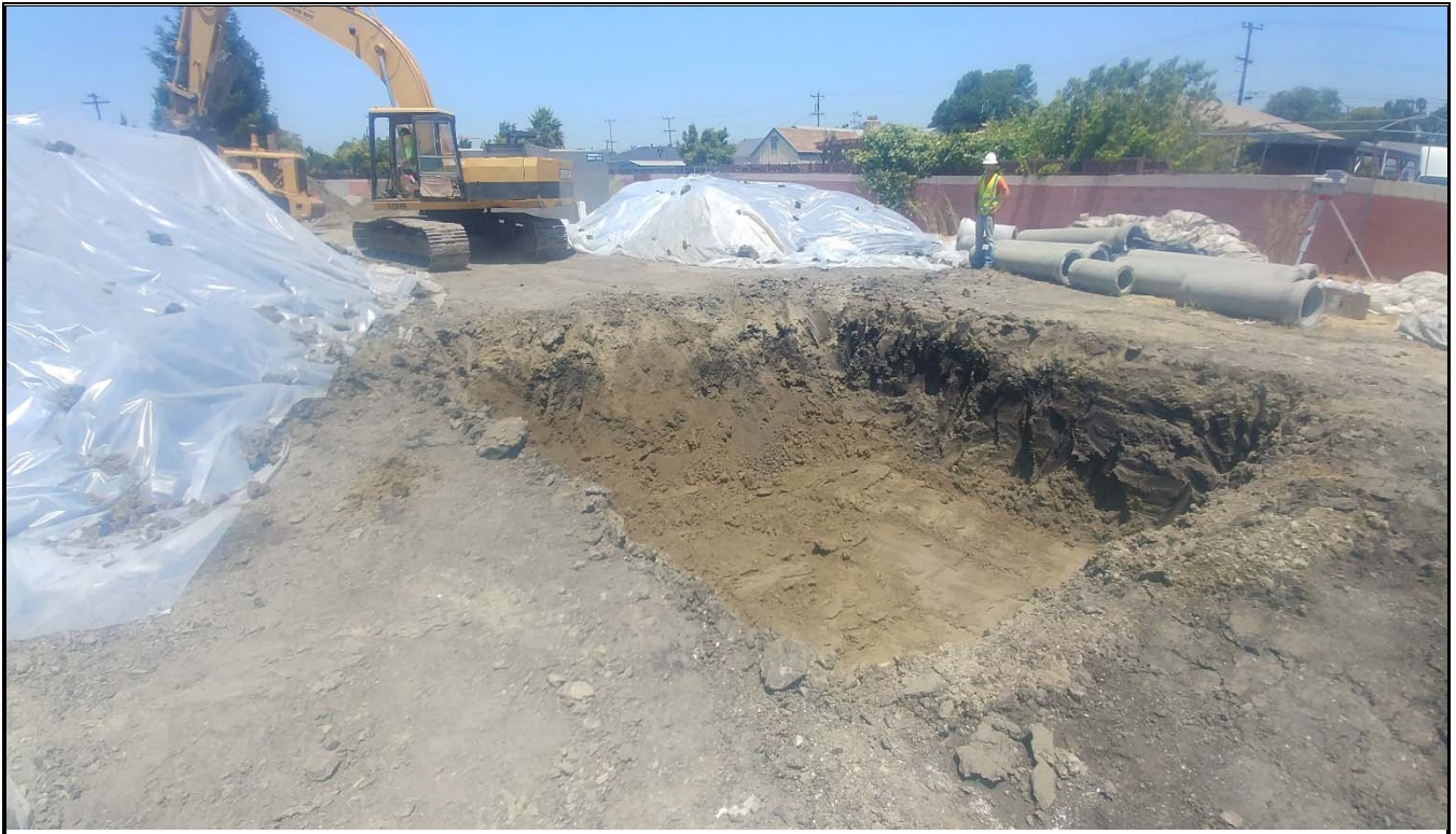
Photo 3. Excavation of ethylbenzene-impacted area (Batch 4).
