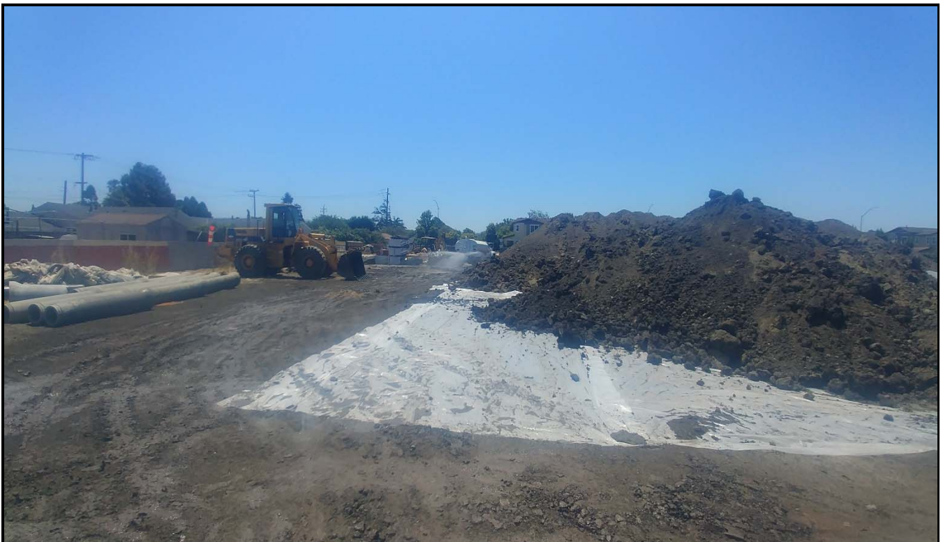
Photo 8. Dust mitigation procedures implemented using water truck to wet roadway.
