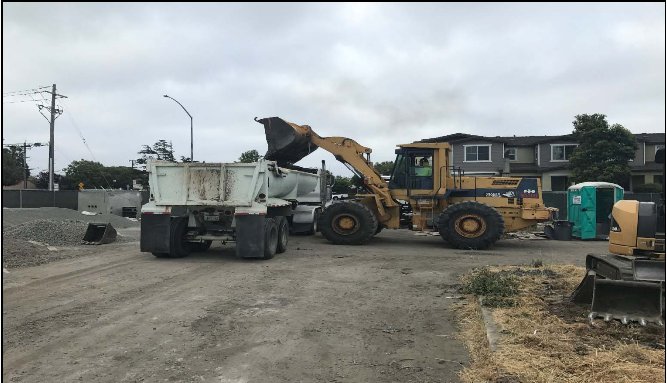
Photo 6. Stockpile soil from Batch 1 being loaded for offsite transport and disposal.
