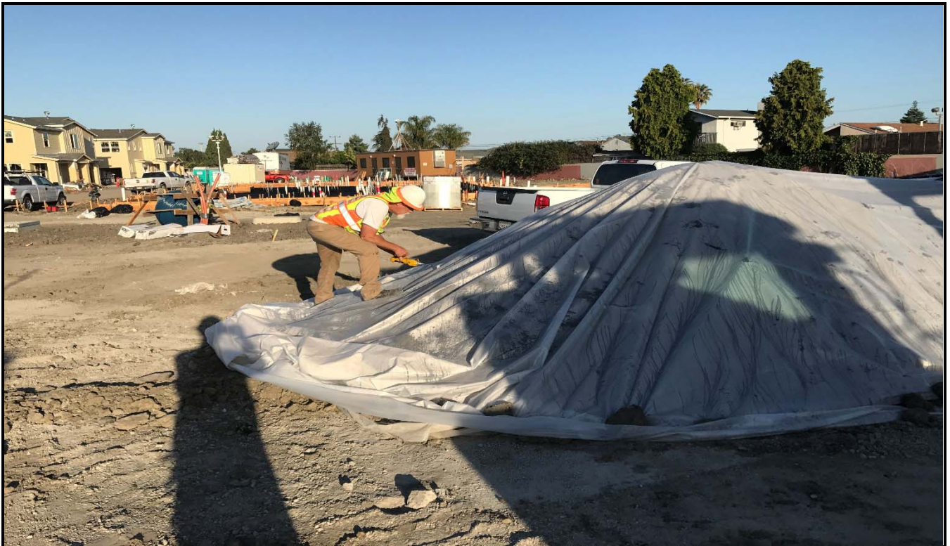
Photo 4. Field screening of soil stockpiles with PID.
