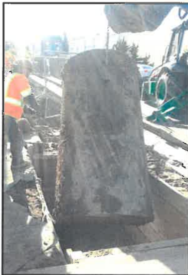
TANK IN EXCAVATION
