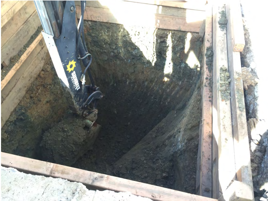
Excavation to 11 feet below ground surface.
