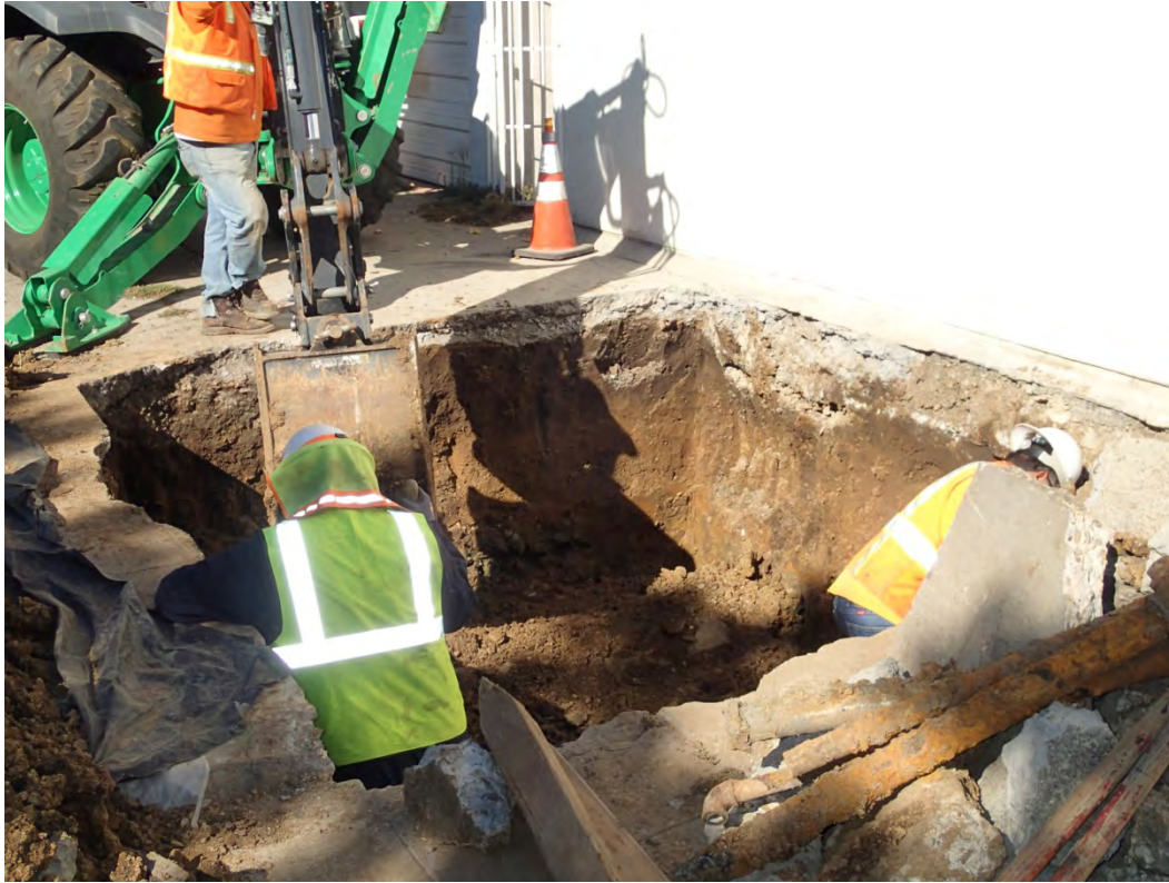
Excavation of overburden.
