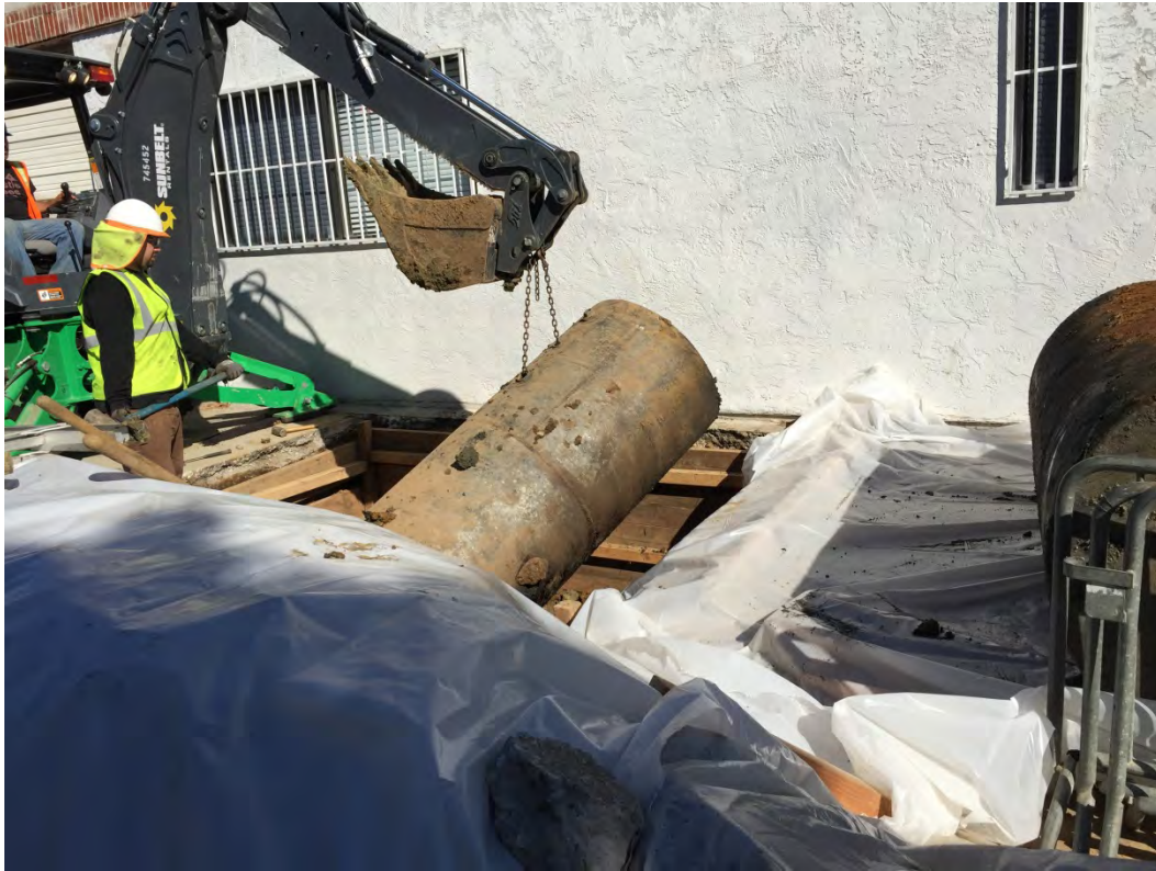
Removal of tanks from excavation.
