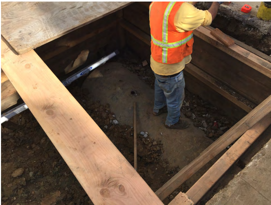
Shoring of excavation sidewalls.
