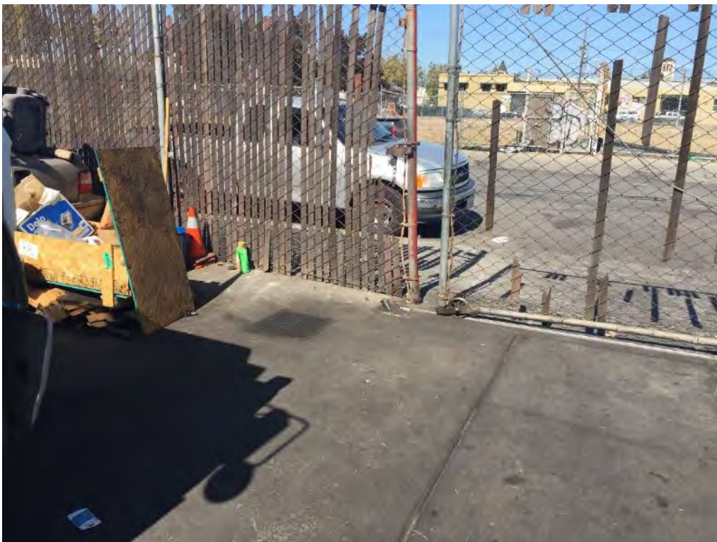
Photograph 15. Storm water drain located in the parking area of the truck repair business.
