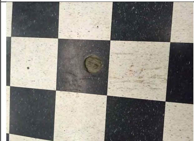
View of surface completion in the craft shop.
