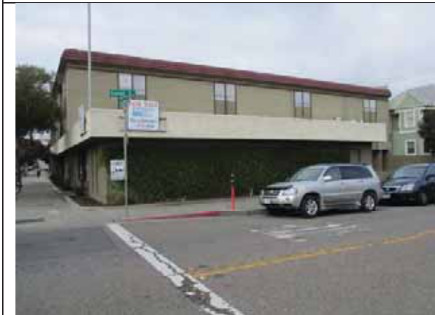
View of the east side of the building.
