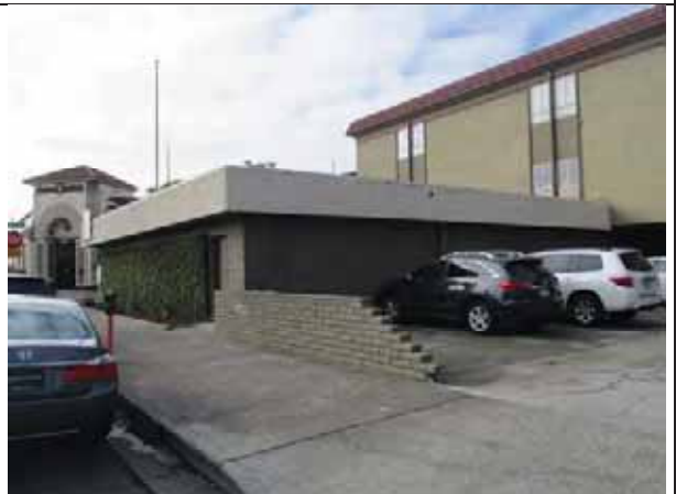
Northeast and southeast sides of the building.
