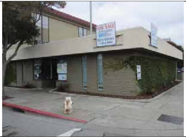
View of the Property from the intersection of Santa Clara Avenue and Everett Street.
