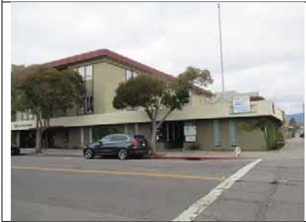
The Property, viewed from Santa Clara Avenue.
