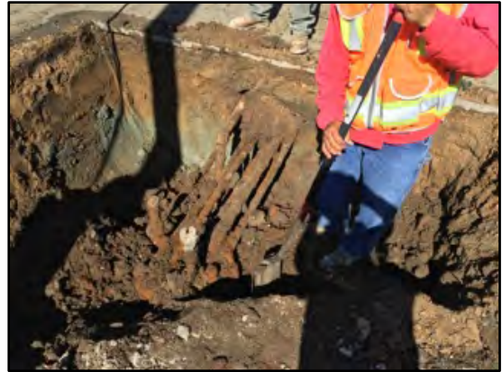
Photograph 20: Additional pipe lines were found running northwest into the subject property from the fifth UST.
