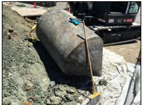
Photograph 12: The fourth UST was found in good condition with no visible holes.
