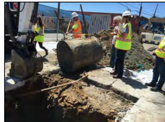
Photograph 4: Residual soil was scraped off of the third UST using a shovel to observe its condition.
