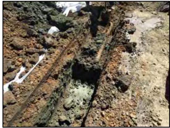
Photograph 26: Trenches were excavated along the piping system for sampling and removal of the piping. Note the shallow olive green soil staining.
