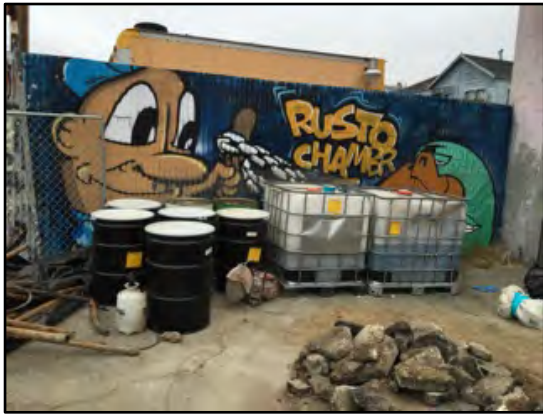
Photograph 25: Tank contents and rinsate were stored on site in DOT-approved 55-gallon drums and 300-gallon totes before being hauled and disposed.
