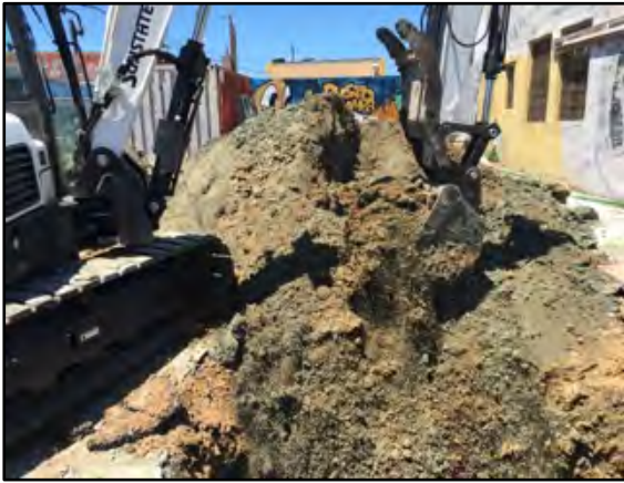
Photograph 15: The third and fourth UST pit was temporarily backfilled using the stockpile soil, which will later be removed during over-excavation.
