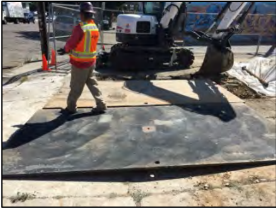
Photograph 7: Trench plates were placed over the open pits for safety until they were backfilled.
