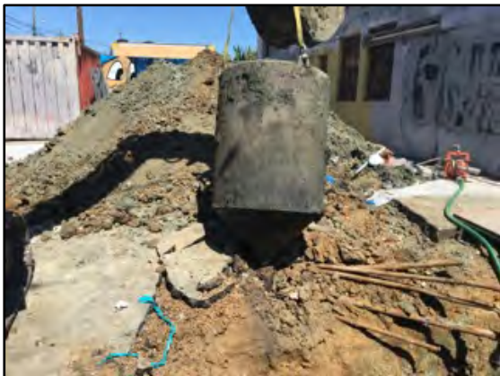
Photograph 11: The fourth UST was removed using the excavator bucket and was found to be an upright, conical tank.
