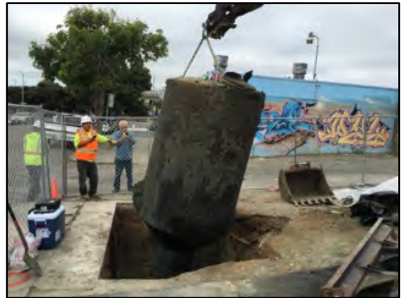
Photograph 22: The fifth UST was removed using the excavator arm.
