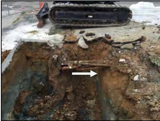
Photograph 9: Multiple pipes were found running northwest (arrow) into the subject property and southwest towards the fifth UST.
