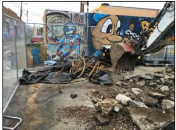
Photograph 28: Approximately 200 ft of piping was removed and stored on a plastic liner before disposal.
