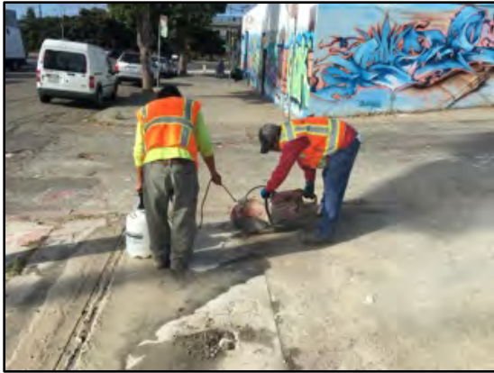
Photograph 19: A saw was used to cut the concrete slab above the fifth UST. The excavation area had previously been cleared for utilities by USA.
