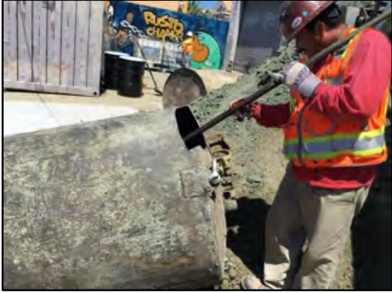
Photograph 13: A hole was cut into the fourth UST and was then triple rinsed by Western Abatement personnel.
