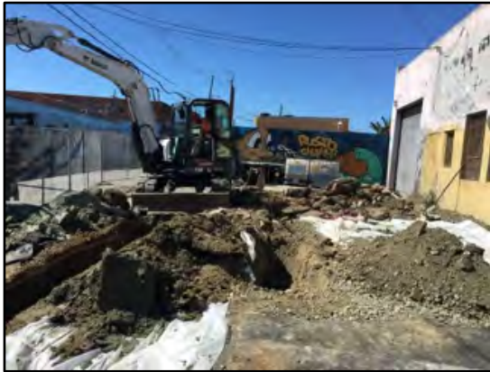
Photograph 27: Trenches running northwest into the property where the pipelines were located.
