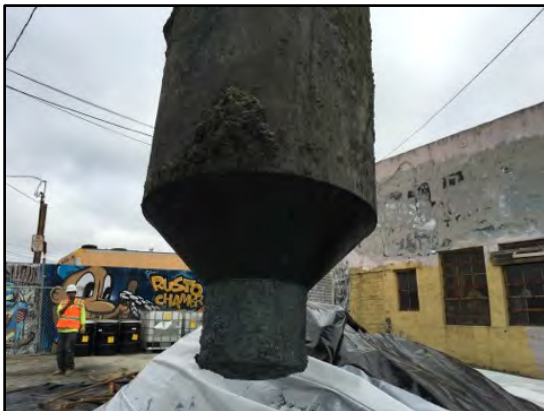
Photograph 23: The fifth UST was found in good condition with no visible holes.
