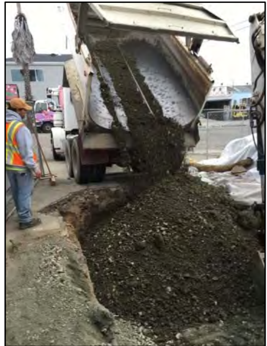
Photograph 14: Clean imported soil was used for backfill.
