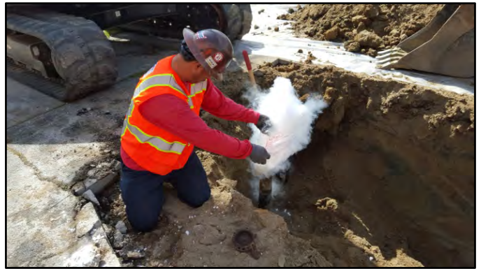
Photograph 2: Dry ice was added to the tank to lower the oxygen level and Lower Explosive Levels (LELs).
