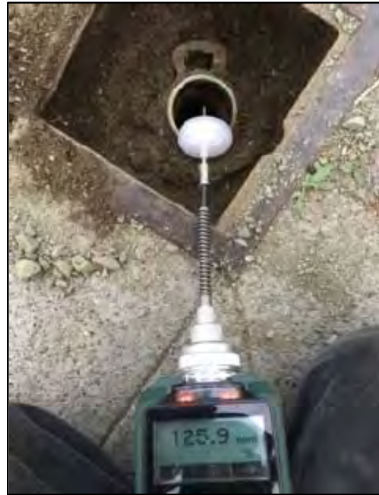
Photograph 16: A third tank was discovered under the sidewalk southeast of the former tank pit. A PID meter was used to measure VOCs at the fill pipe of the third tank.
