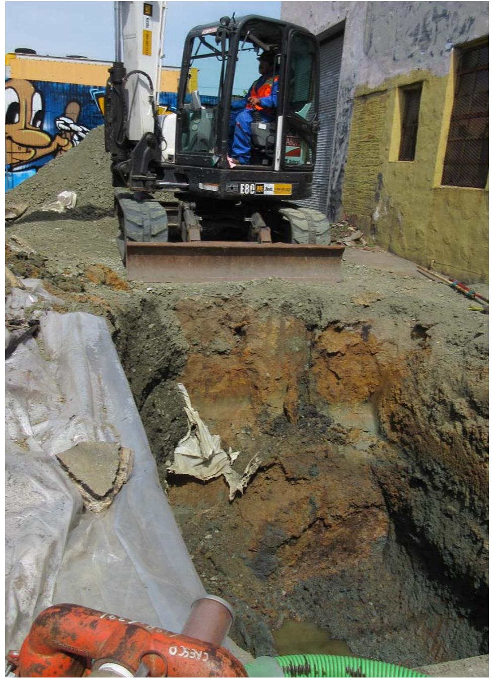
1647 International Blvd B Jakub, April 7, 2016 Tank pit
