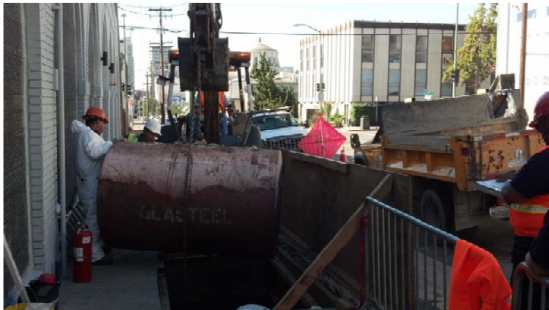
TANK REMOVAL IN PROCESS
