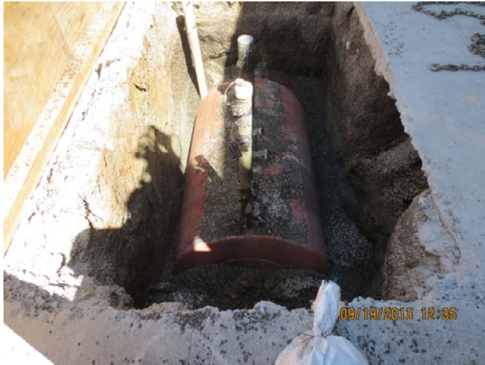
UST READY TO BE REMOVED FROM EXCAVATION
