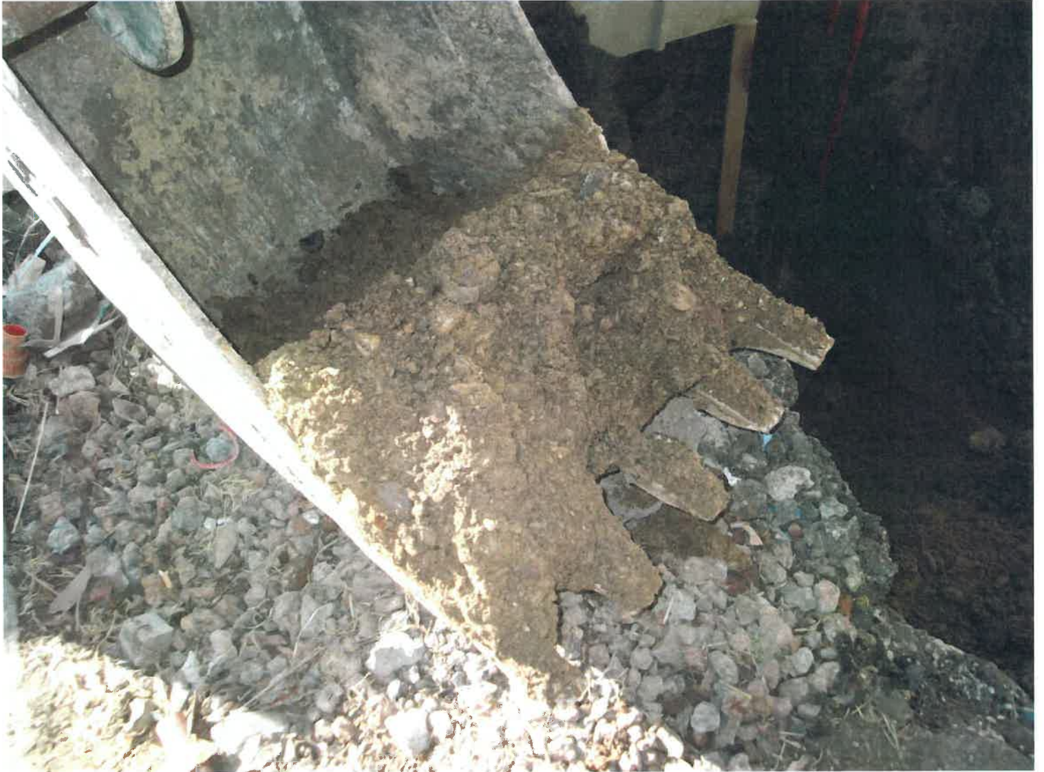
Image # 7 Soil in backhoe bucket from UST soil sample collection depth.
