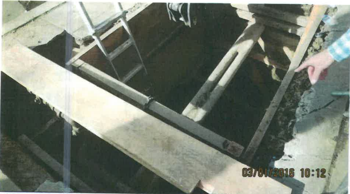
DESCRIPTION: TANK PIT Photo # 1 of 43
