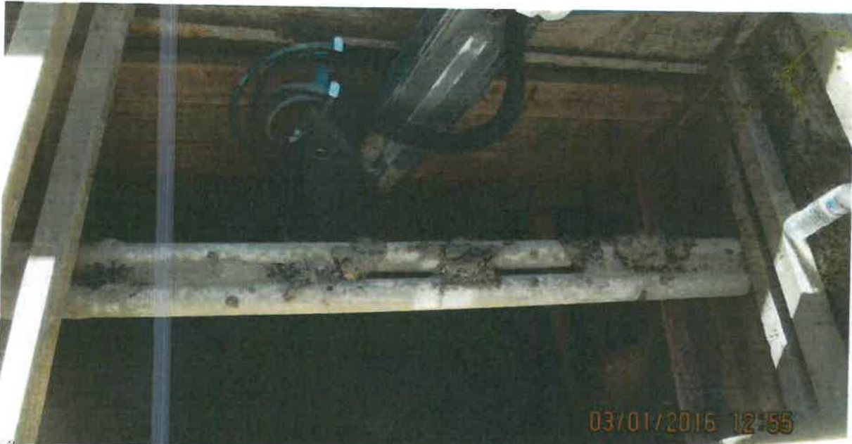
DESCRIPTION: OVER-EXCAVATING PROCESS Photo # 25 of 43
