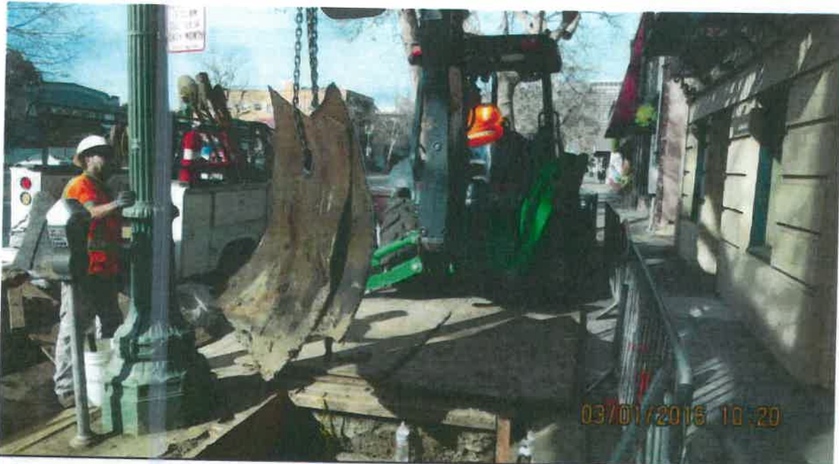
DESCRIPTION: REMOVAL OF CUT PORTIONS OF TANK
