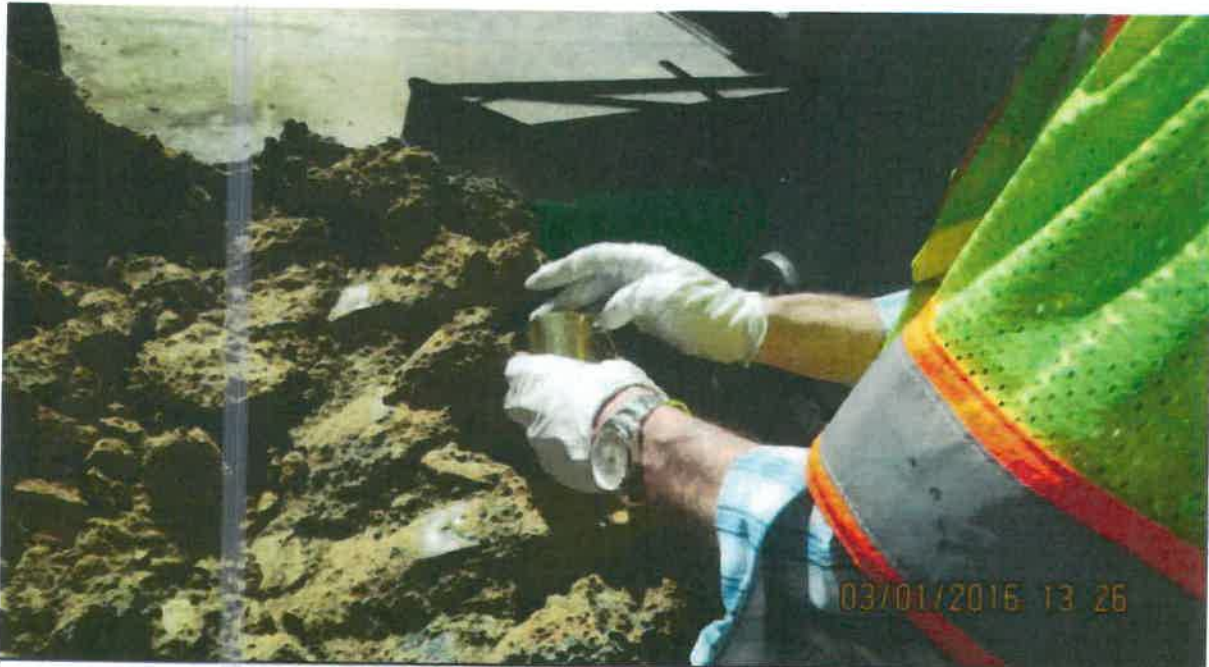
DESCRIPTION: SOIL SAMPLE COLLECTED AFTER OVER-EXCAVATING
