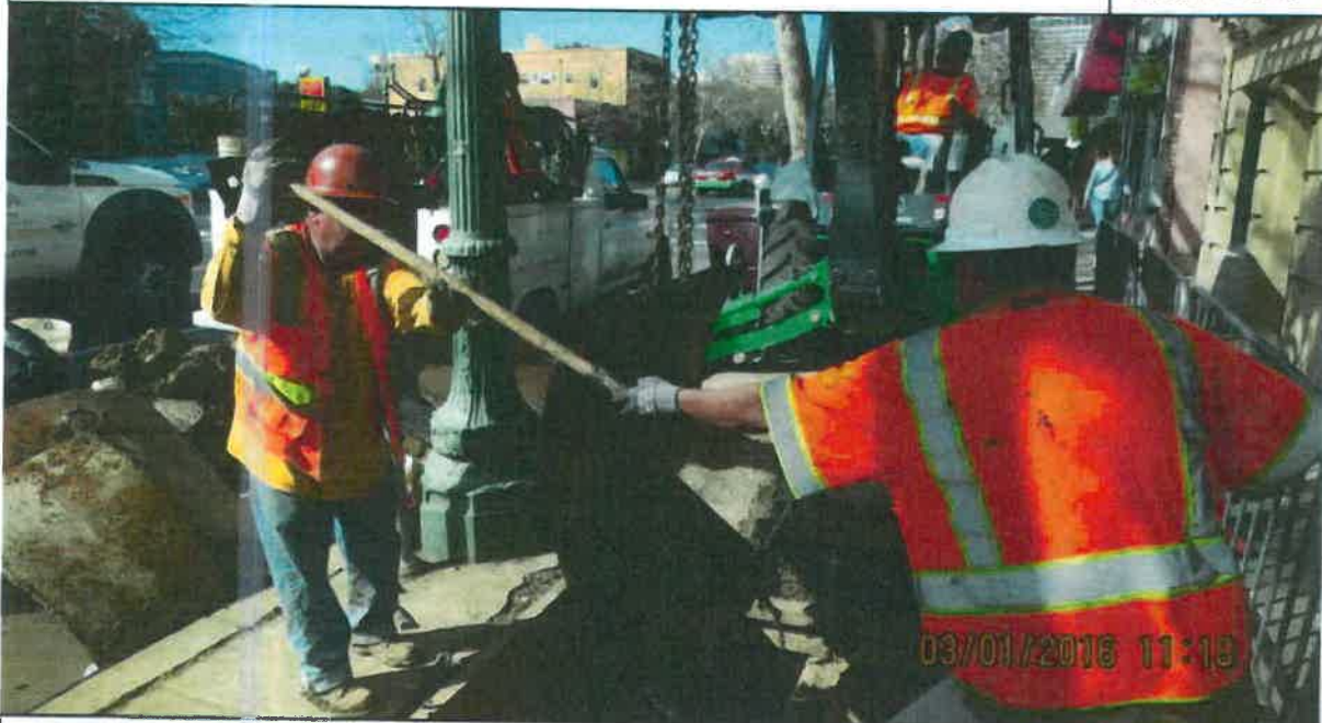
DESCRIPTION: REMOVING MORE OF THE TANK
