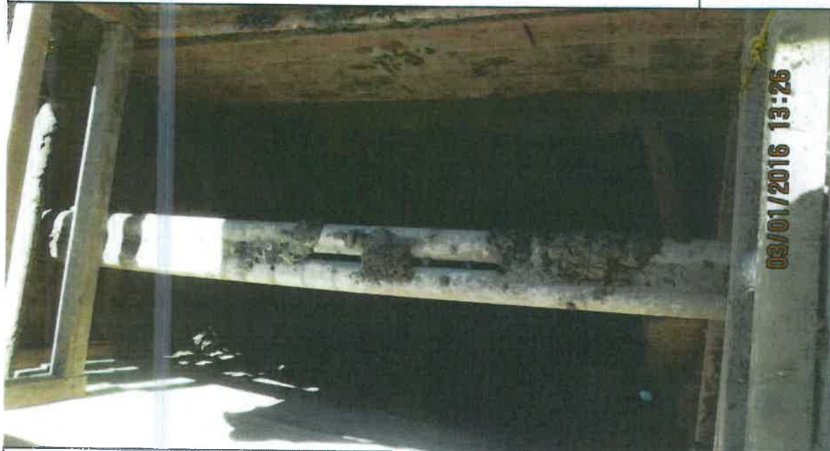
DESCRIPTION: VIEW OF TANK PIT DURING OVER-EXCAVATING PROCESS
