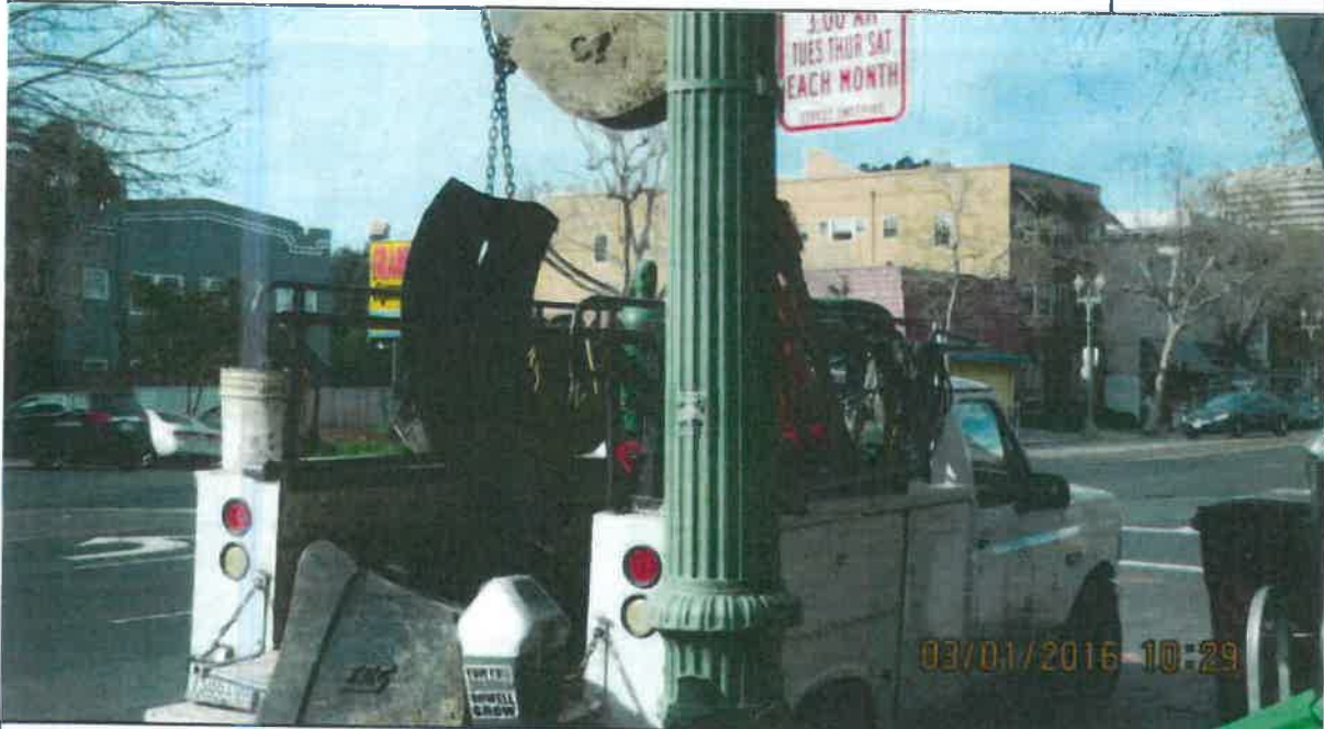
DESCRIPTION: PORTION OF TANK REMOVAL
