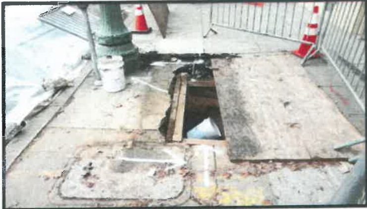
TANK IN EXCAVATION
