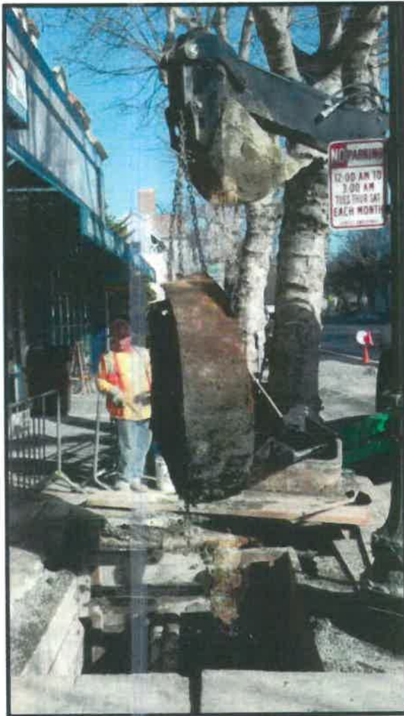
TANK REMOVAL IN PROGRESS
