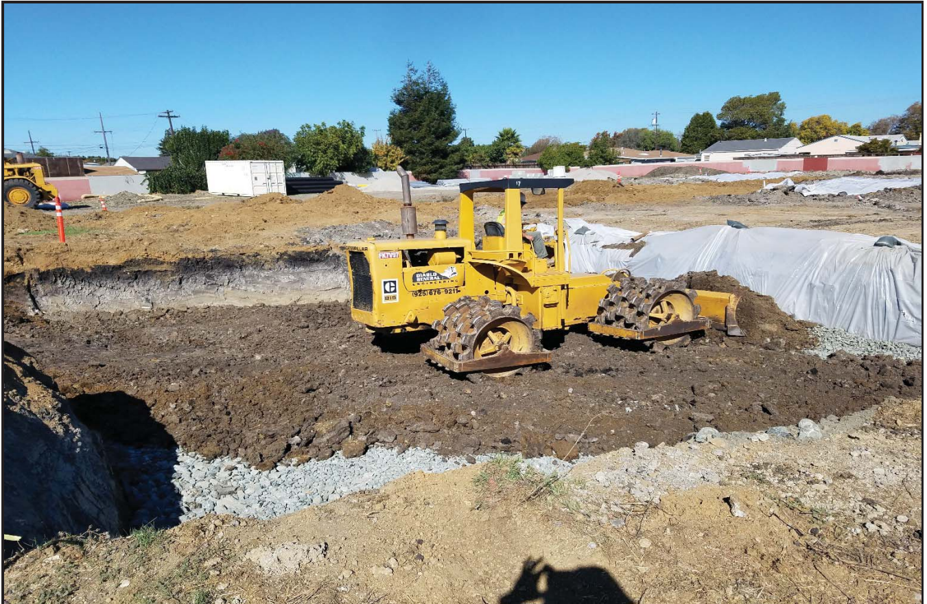
Photo 4. Backfilling and compaction of PTN excavation
