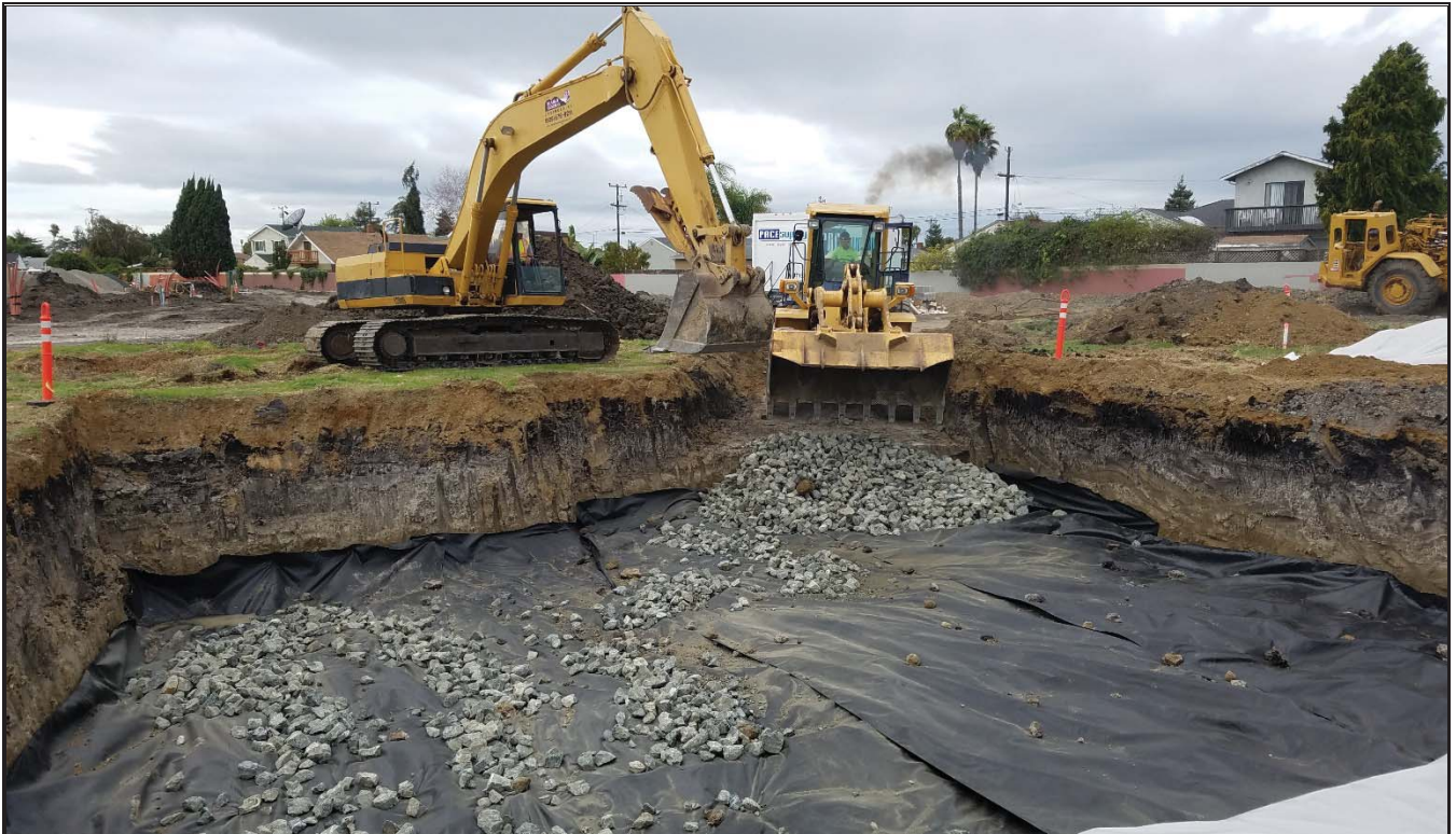
Photo 3. Placement of imported gravel in bottom of PTN excavation
