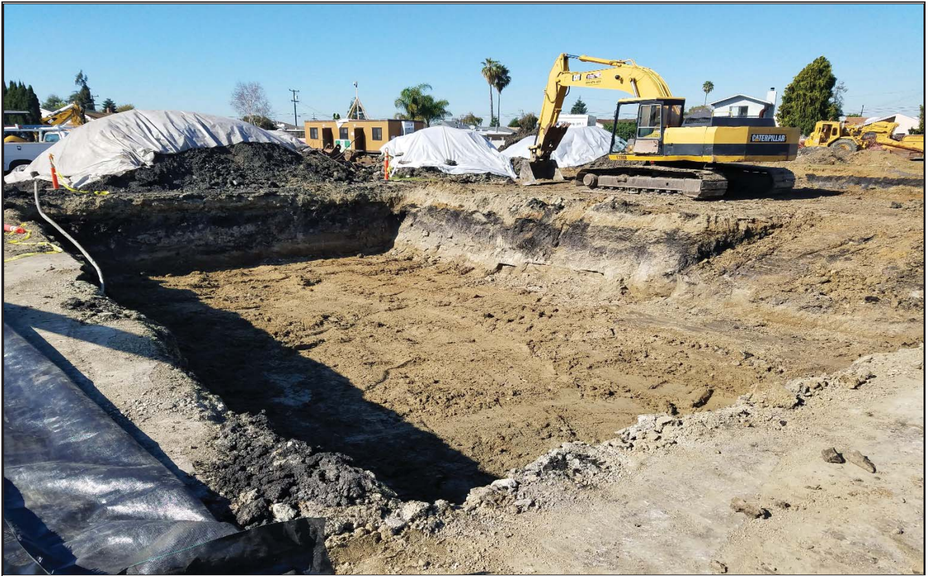
Photo 5. PTS excavation area
