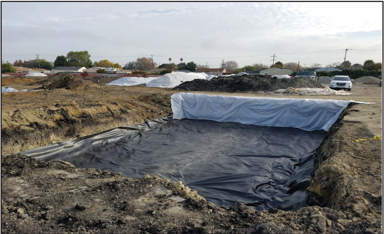
Photo 6. Bottom geotextile fabric and plastic vapor barrier in PTS excavation
