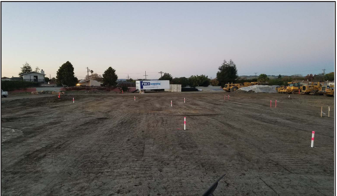
Photo 8. Completed excavations and soil gas probes with protective monument casings
