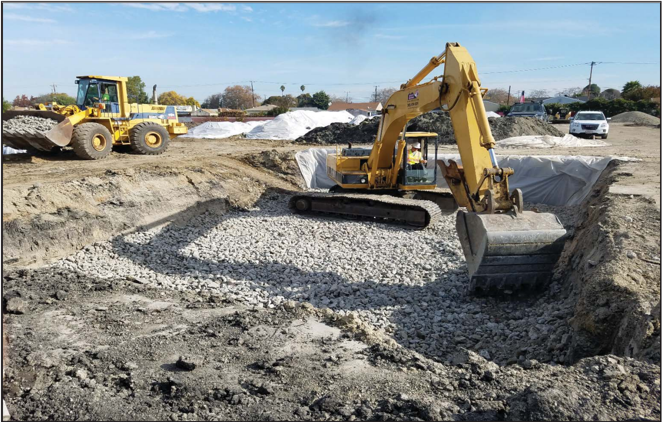
Photo 7. Placement of imported gravel in bottom of PTS excavation
