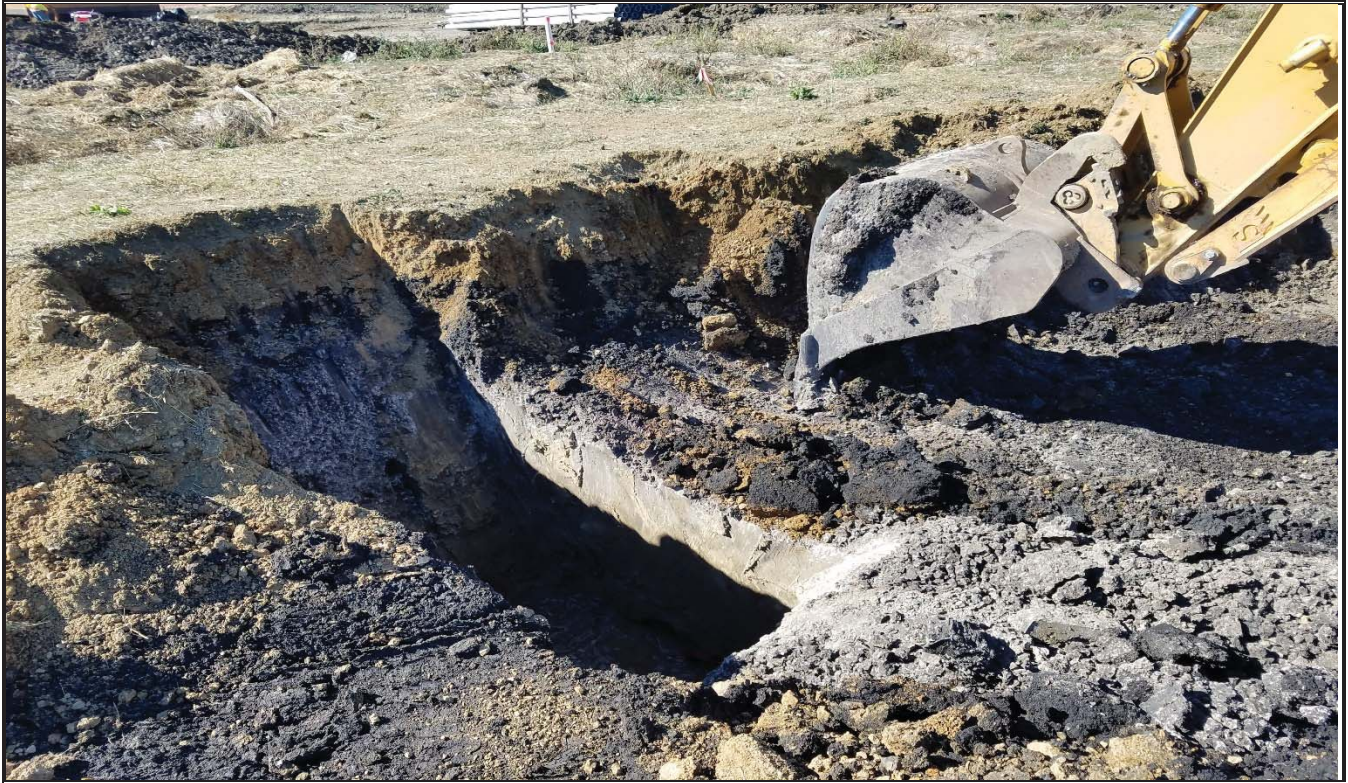
Photo 1. Test pit within Pilot Study Excavation area
