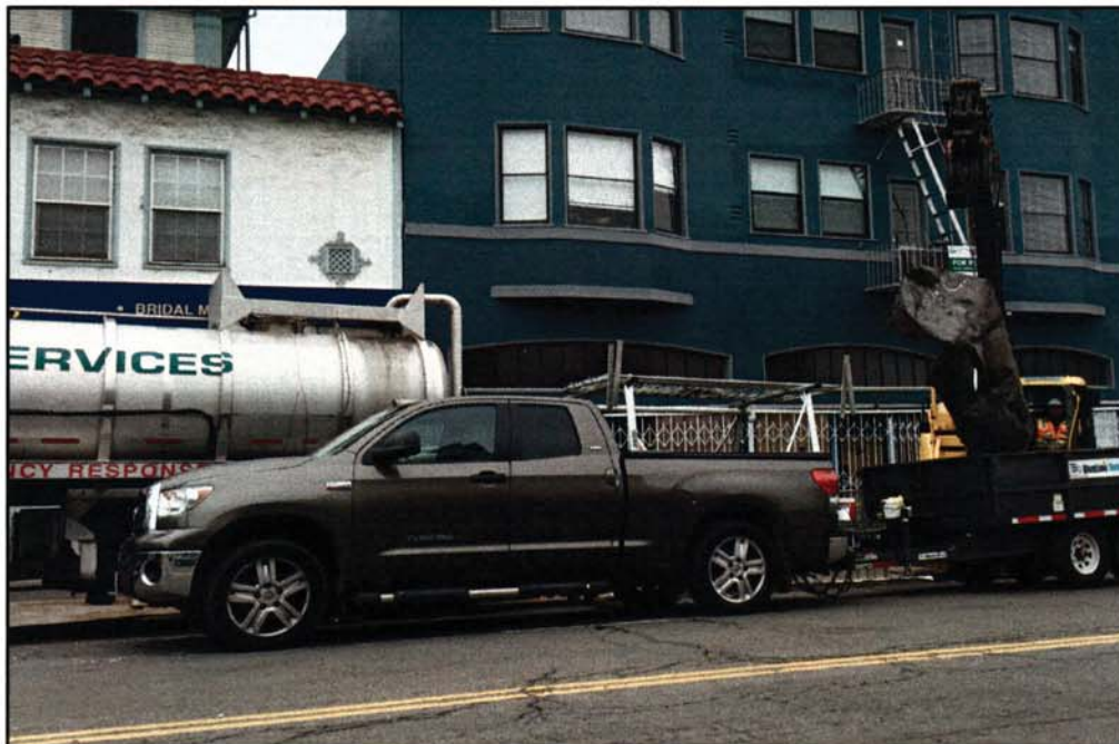
Loading UST for transport to metal recycling facility.
