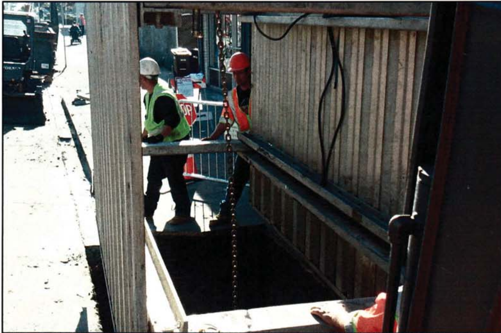
Trenchshield is installed to support excavation due to groundwater intrusion.
