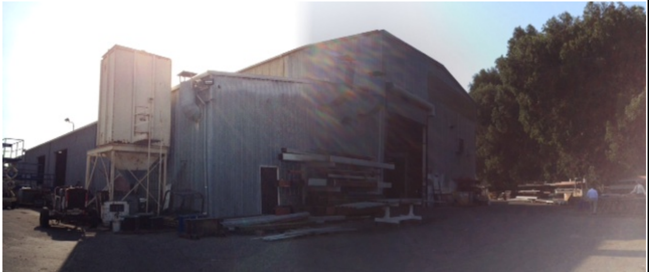
Photo 4: Subject Site (Facing Southeast) Partial Two-Story Commercial Office/Warehouse Building
