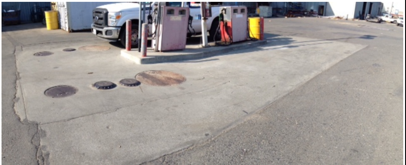
Photo 22: Subject Site (Facing Southwest) Fuel Dispensers and Underground Storage Tanks
