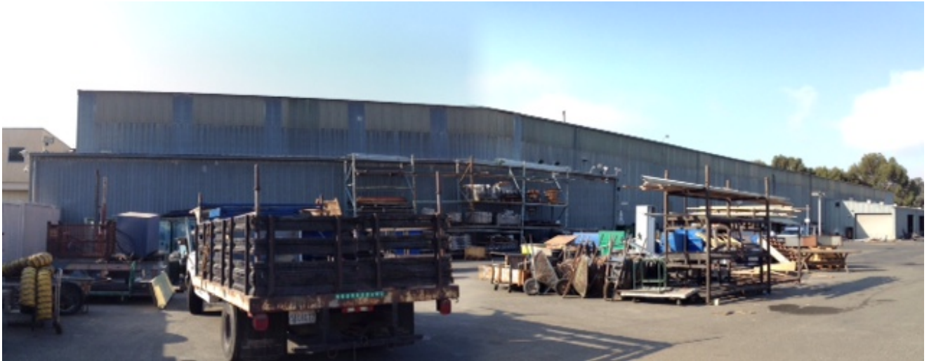
Photo 3: Subject Site (Facing South) Partial Two-Story Commercial Office/Warehouse Building
