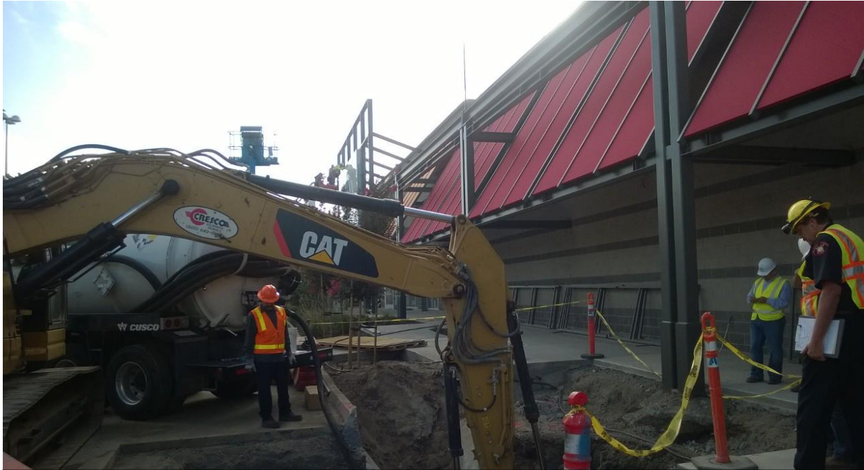
DESCRIPTION: EXCAVATION CONTINUING – LOCATION IN RELATION TO BUILDING AND PILLAR
