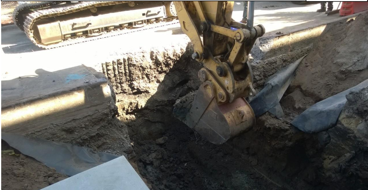
DESCRIPTION: SOIL SAMPLE COLLECTED FROM SOUTH SIDE OF EXCAVATION UNDER TANK
