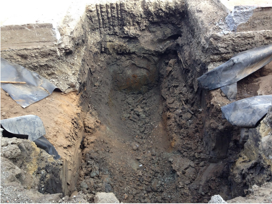
Photograph 5. Excavation post UST removal.
