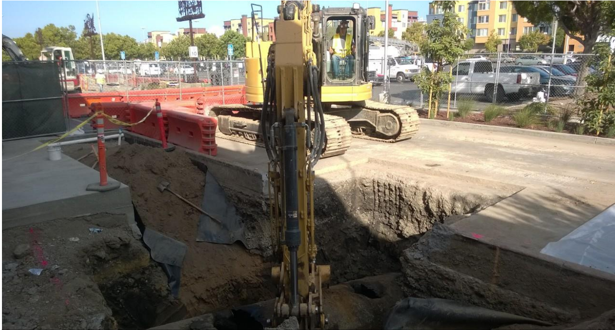
DESCRIPTION: UST BEING REMOVED Photo # 7 of 25
