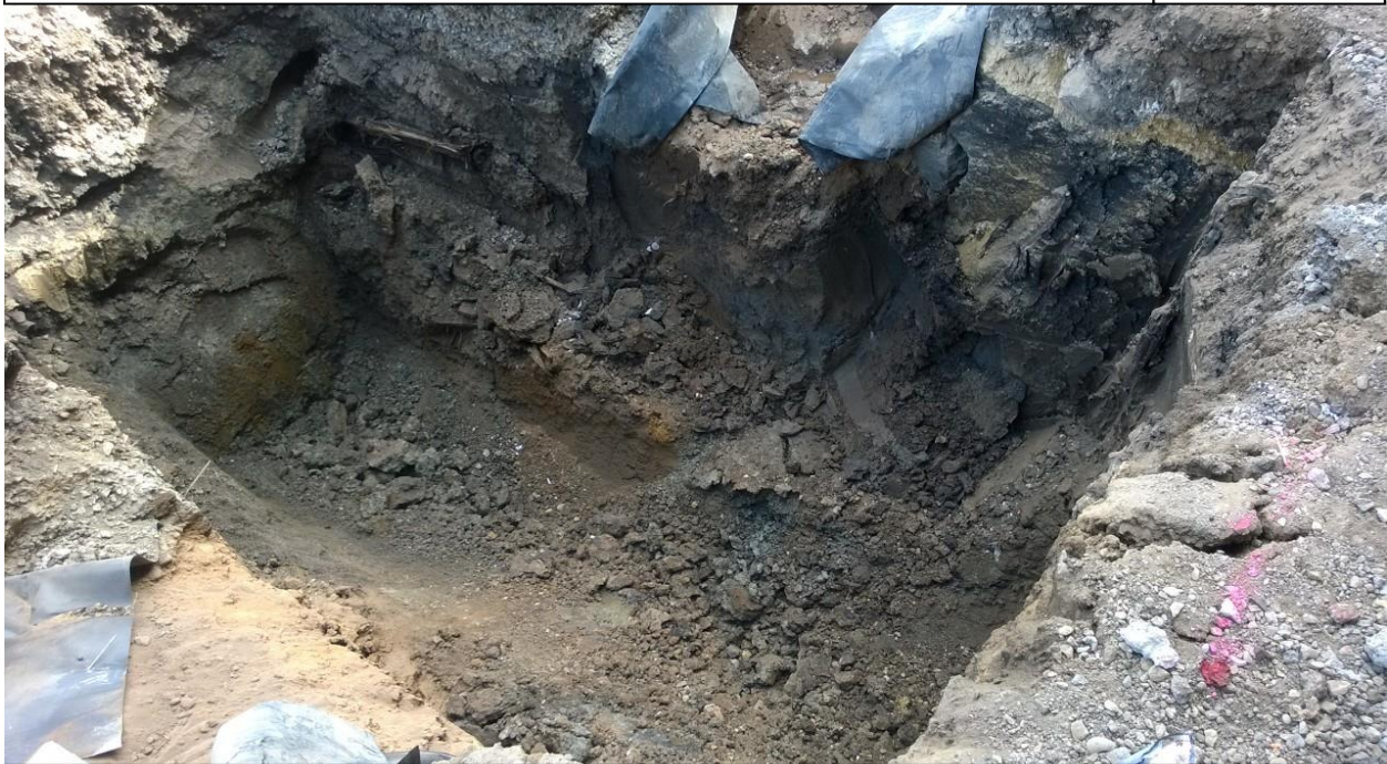
DESCRIPTION: EXCAVATION Photo # 14 of 25
