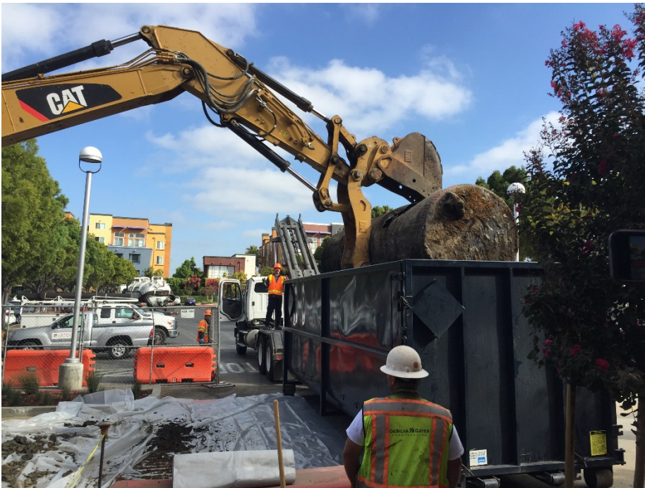
Photograph 4. Placement of UST into bin for off-Site disposal.
