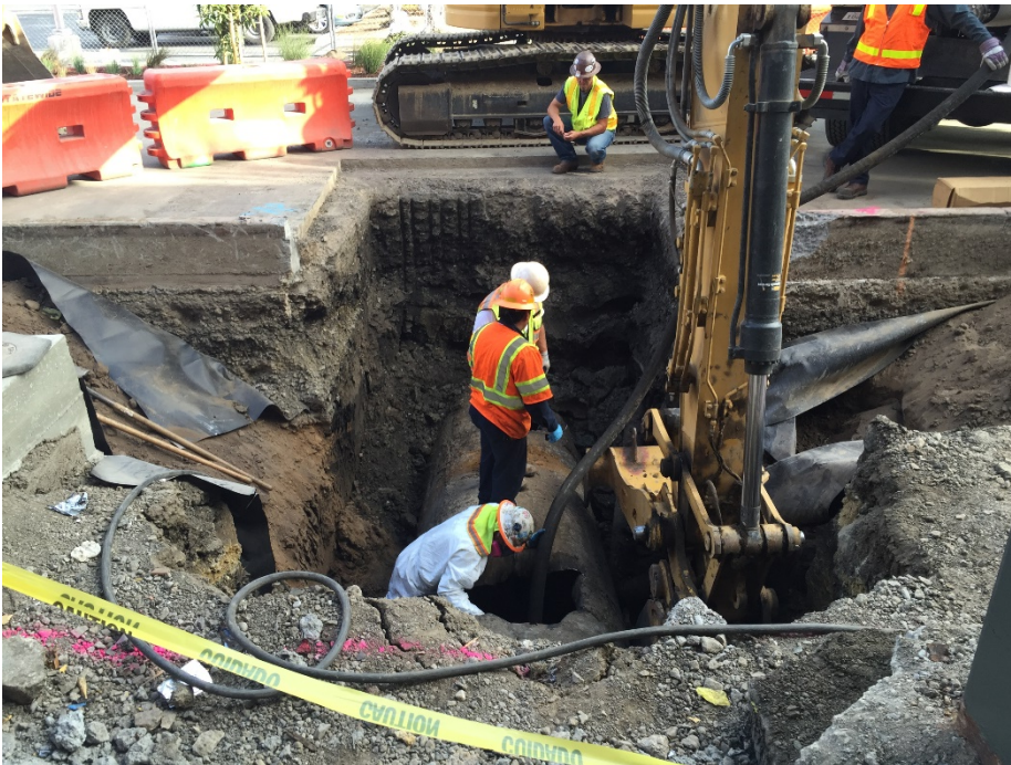
Photograph 2. Pumping of residual fluid from UST.
