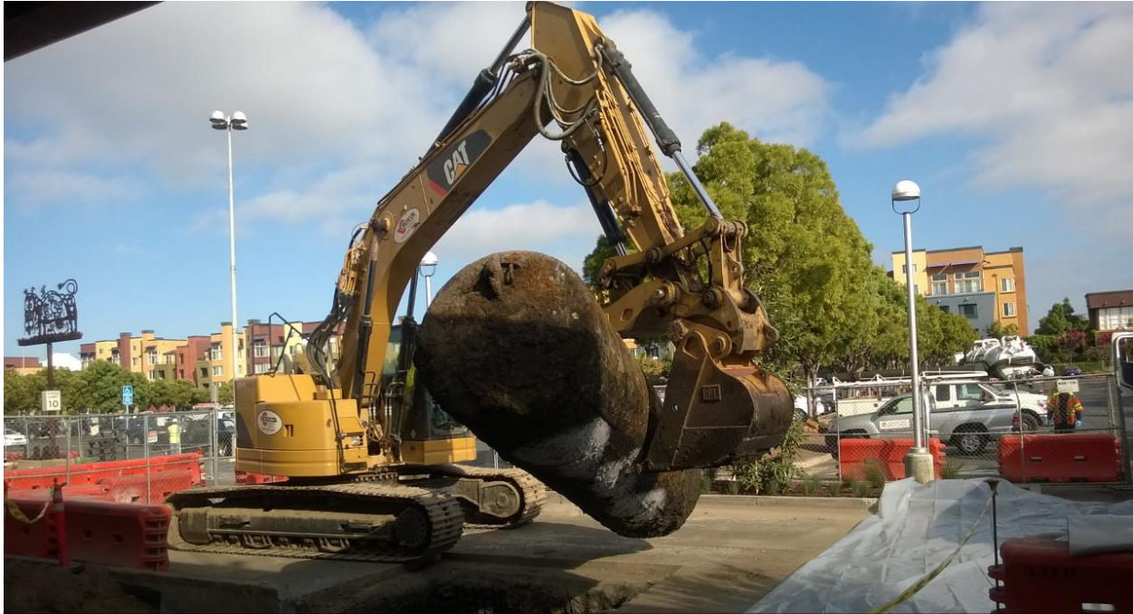
DESCRIPTION: UST BEING REMOVED
