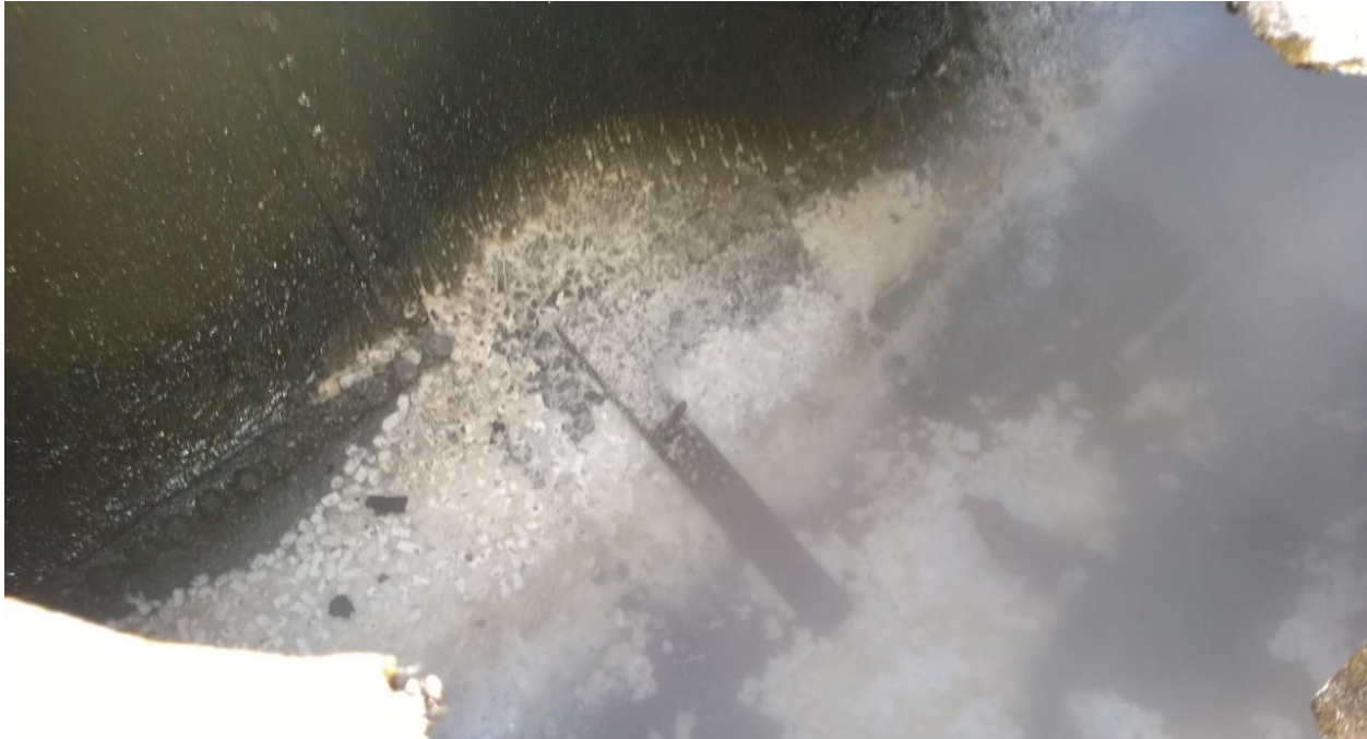
DESCRIPTION: VIEW OF DRY ICE PRESENT IN UST Photo # 13 of 25
