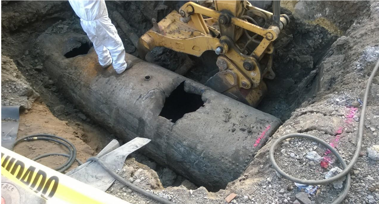
DESCRIPTION: EXCAVATION CONTINUING
