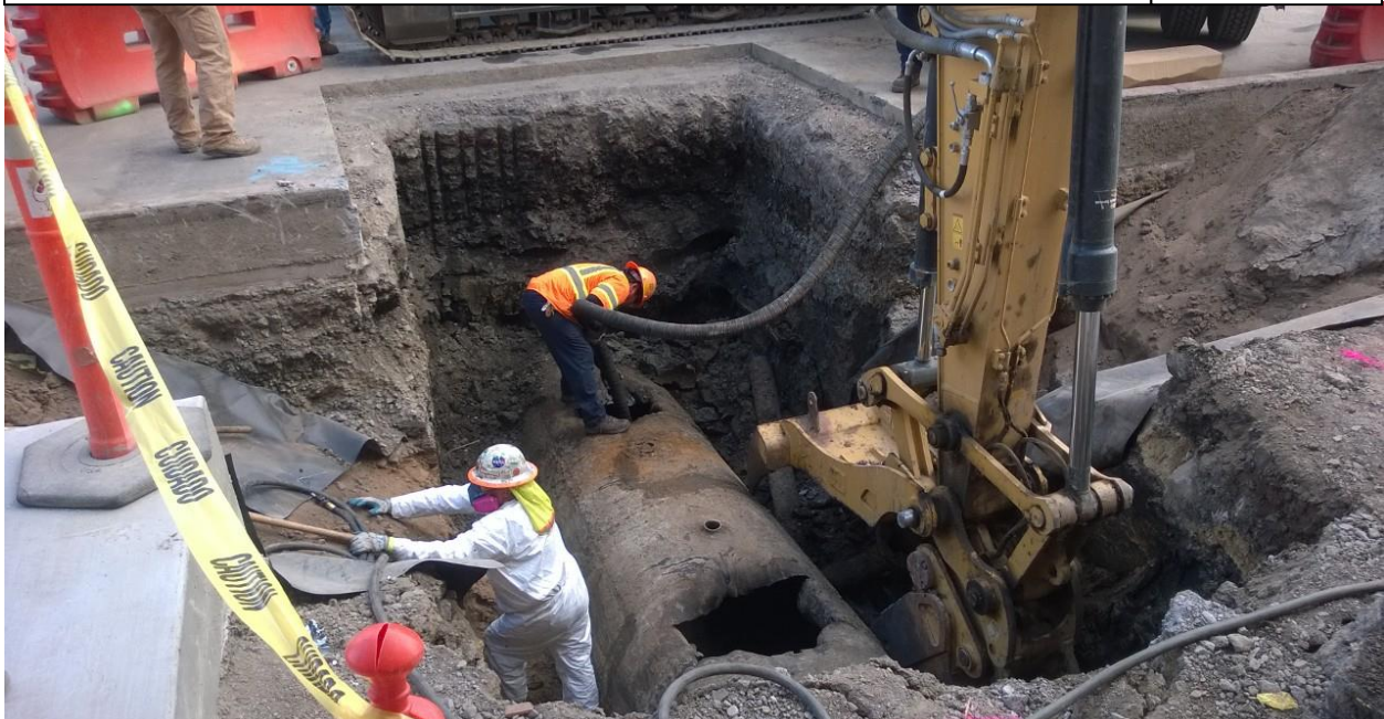
DESCRIPTION: EXCAVATION – RESIDUAL LIQUID BEING PUMPED OUT.
