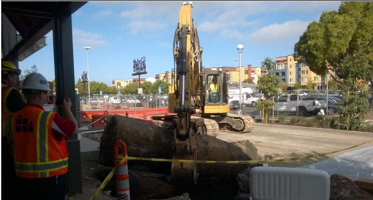
DESCRIPTION: UST BEING REMOVED Photo # 8 of 25
