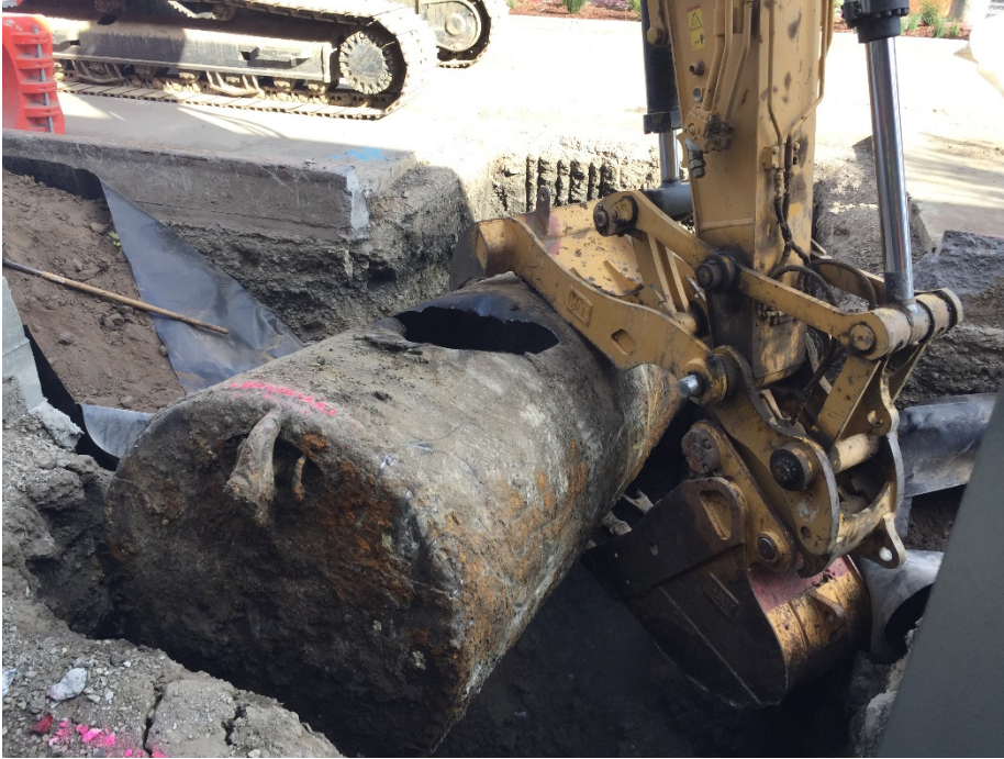
Photograph 3. Removal of UST from excavation.
