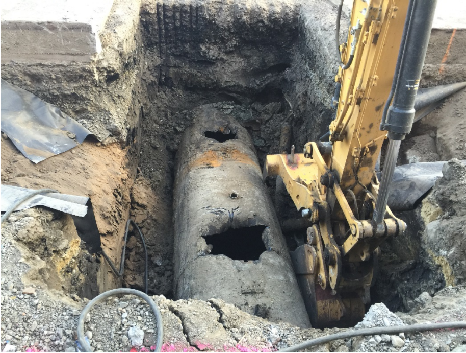
Photograph 1. Excavation of soil adjacent to the diesel UST.
