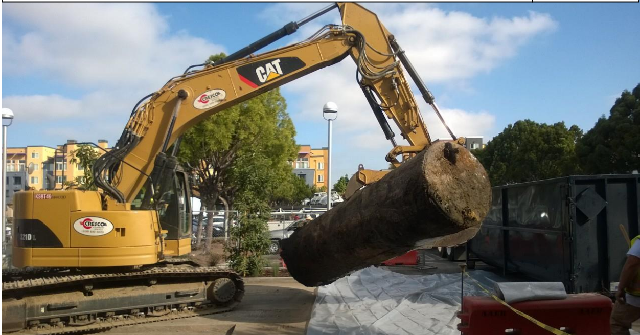
DESCRIPTION: UST BEING REMOVED – NO OBSERVED LEAKING
