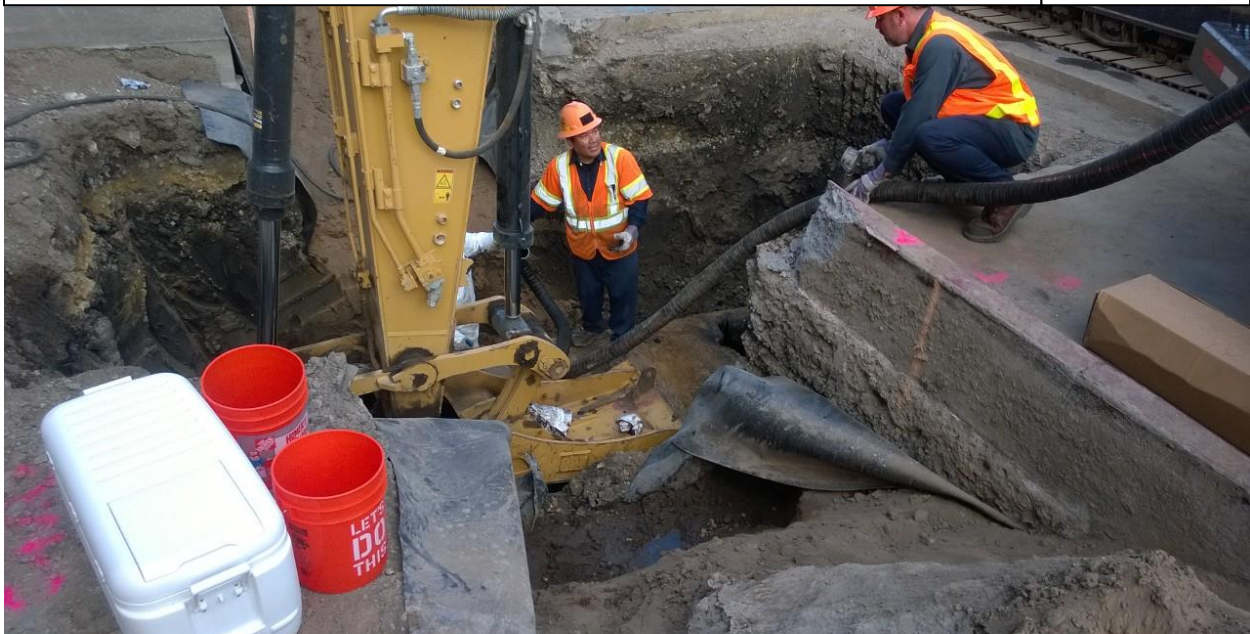
DESCRIPTION: EXCAVATION CONTINUING – DRY ICE PLACED NEAR EXCAVATION
