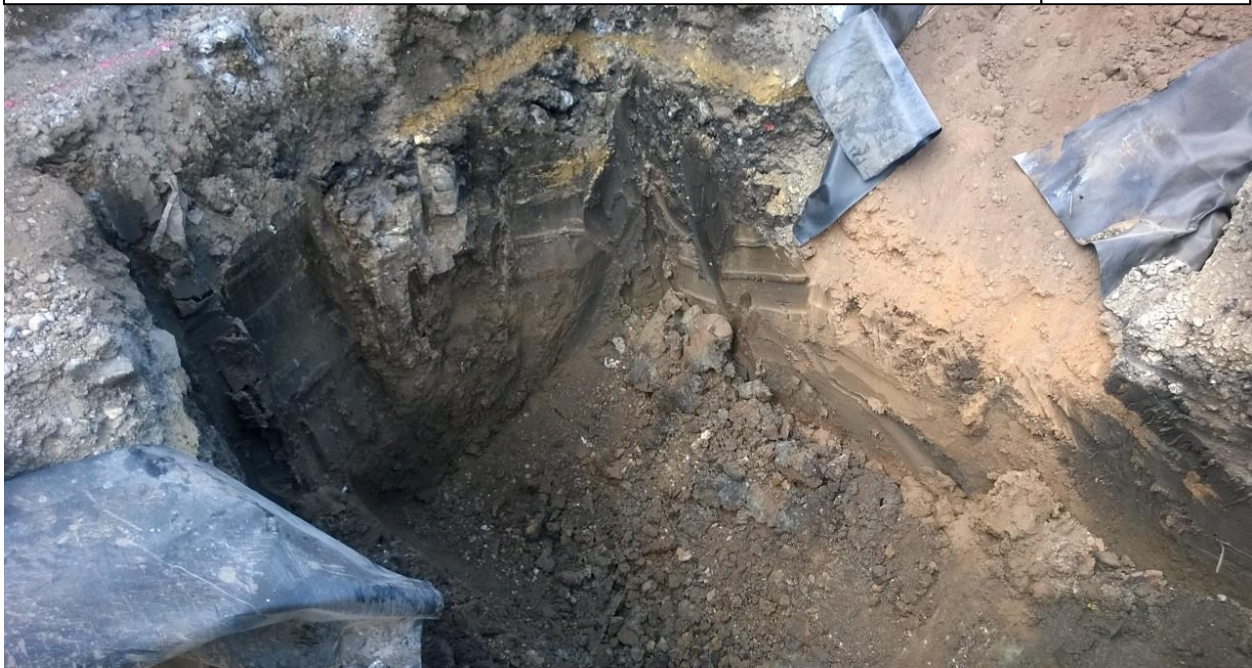
DESCRIPTION: VIEW OF EXCAVATION
