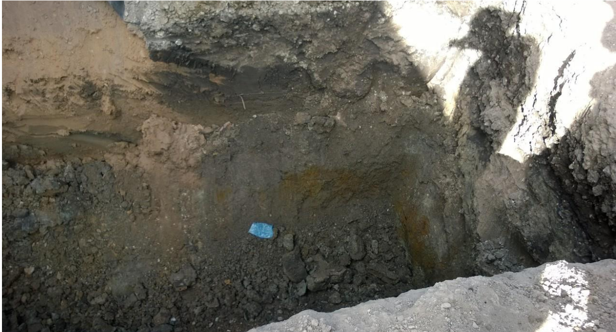
DESCRIPTION: VIEW OF EXCAVATION
