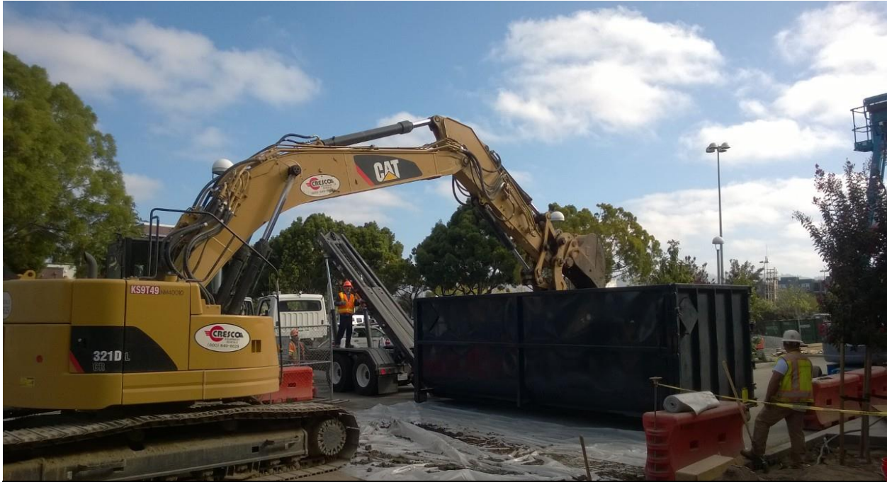
DESCRIPTION: TANK PLACED IN BIN.
