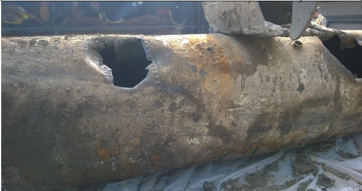
DESCRIPTION: CHECKING REMOVED UST FOR HOLES OR CRACKS.
