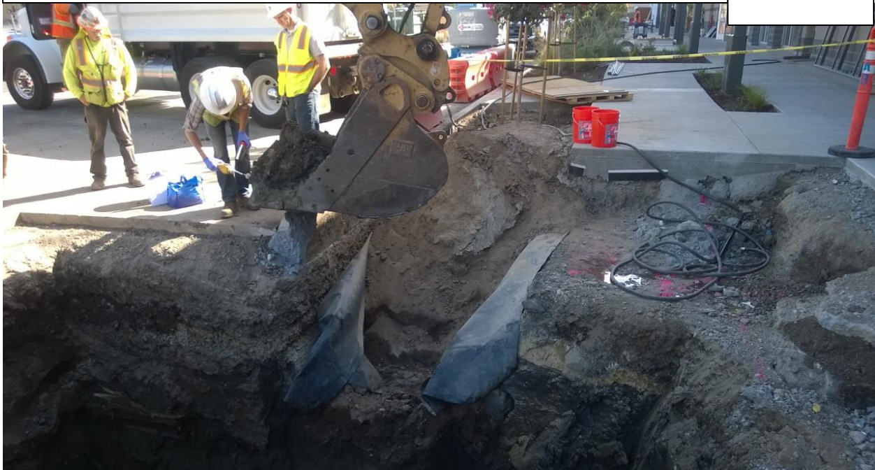
DESCRIPTION: SOIL SAMPLE COLLECTED FROM SOUTH SIDE OF EXCAVATION UNDER TANK
