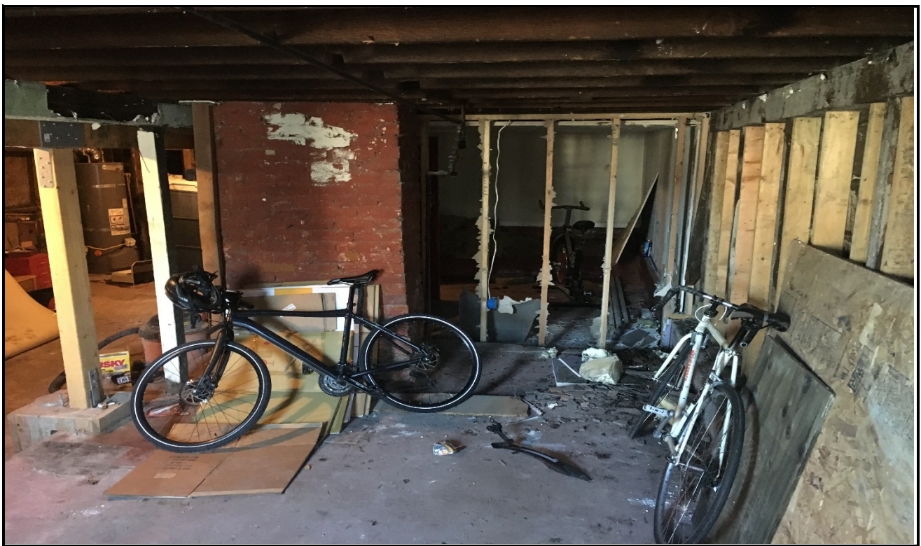
Photo 2. Interior of basement for 2006 Myrtle Street, looking towards to east.
