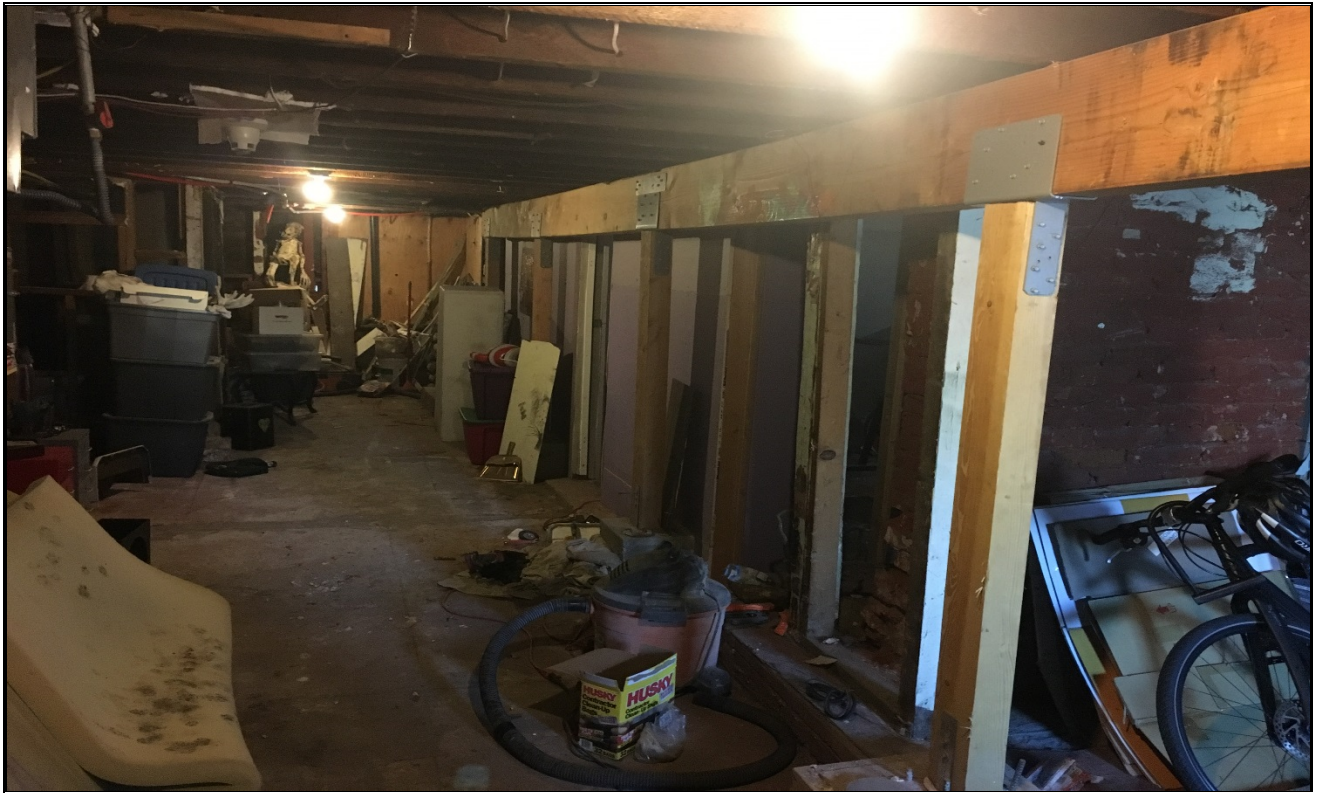
Photo 3. Interior of basement for 2006 Myrtle Street, looking towards the east.
