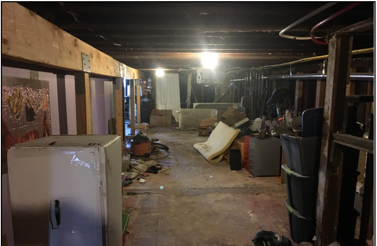
Photo 4. Interior of basement for 2006 Myrtle Street, looking towards the west.
