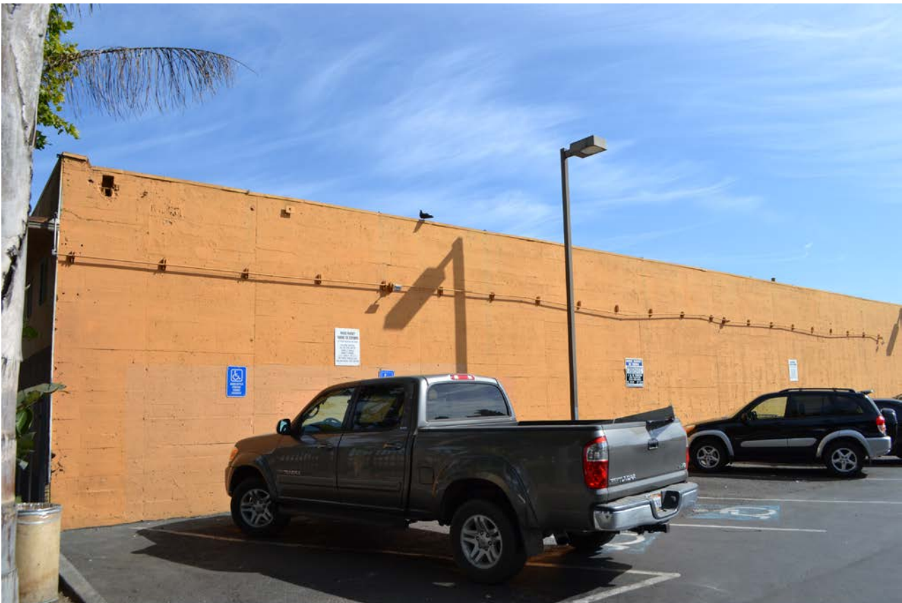
Photo 10: The southern end of the property at 9500 International Blvd. across the parking from a Mexican supermarket MiTierra.
