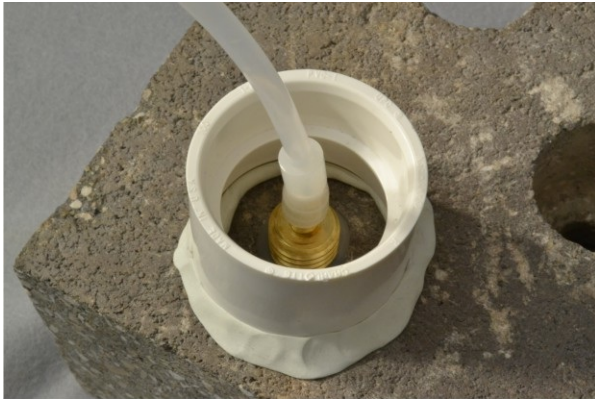
Figure 6. Water dam used for leak detection.
