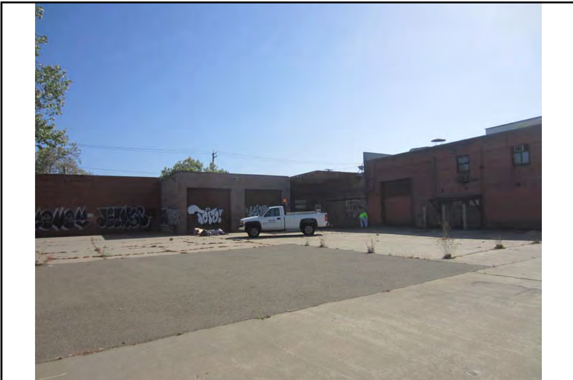
Photograph: 2 General view of the subject property, with asphalt patch from former USTs and site buildings in background.
