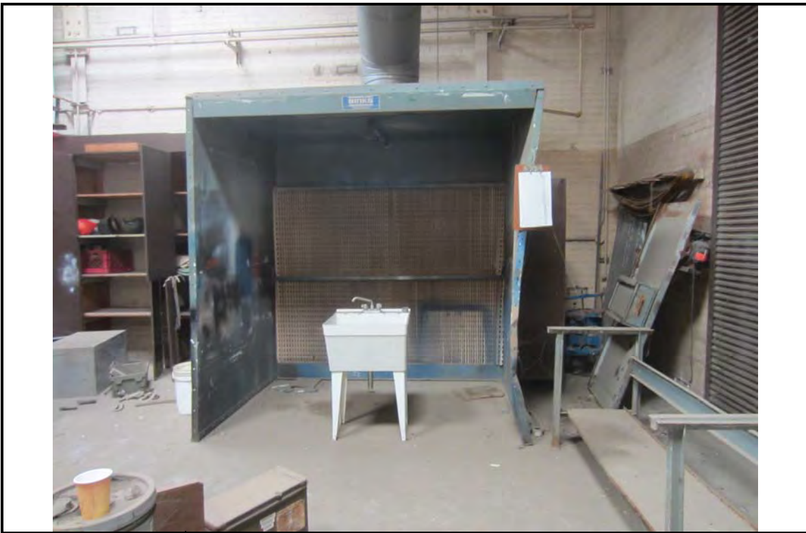
Photograph: 5 | View of paint booth in Building 1.
