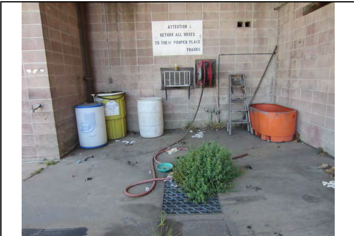
Photograph: 4 | View of the former vehicle wash area with associated sump.
