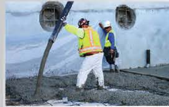
Concrete is placed directly onto the completed Geo-Seal system
