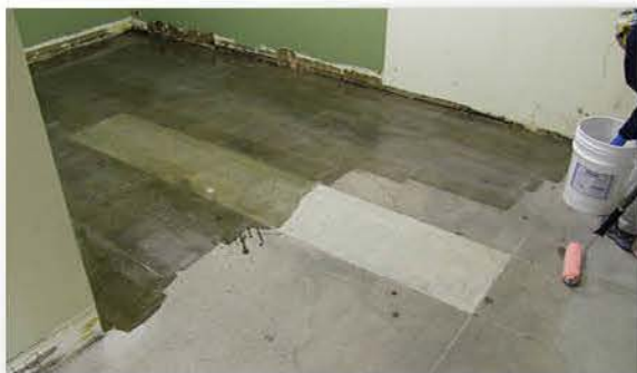
Retro-Coat PRIMER is applied to the concrete surface as final preparation
