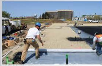
Geo-Seal BASE is a composite sheet material comprised of HDPE and non-woven geotextile
