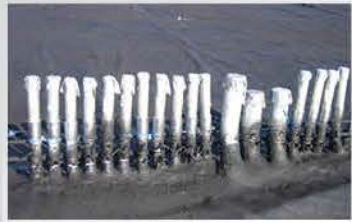
Penetrations are sealed individually
