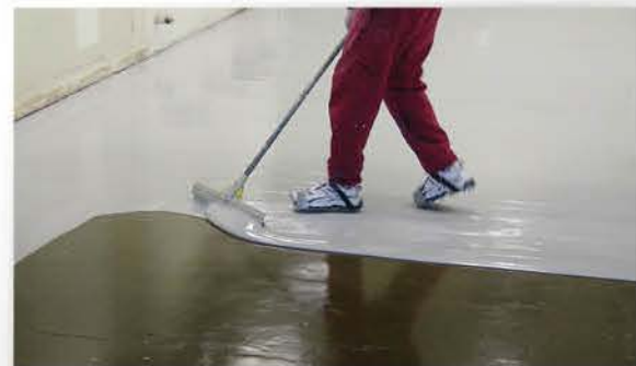
Retro-Coat is applied to a nominal thickness of 20 dry mils
