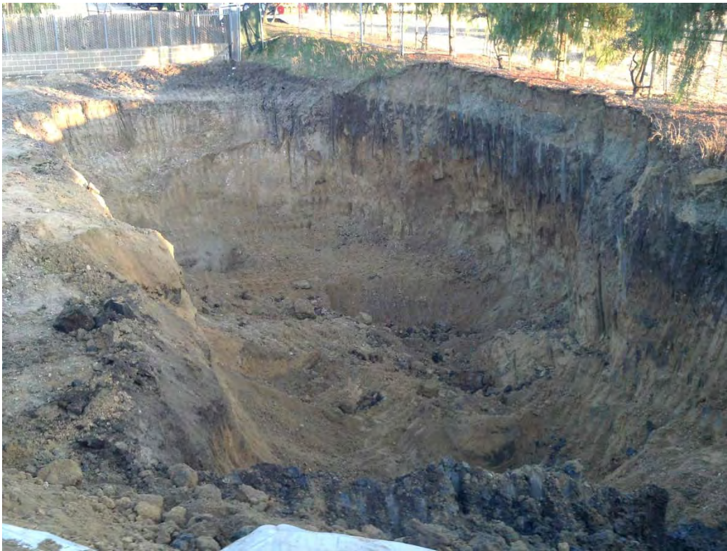
Photograph 2: Facing east at the excavation as activities continued to the west.
