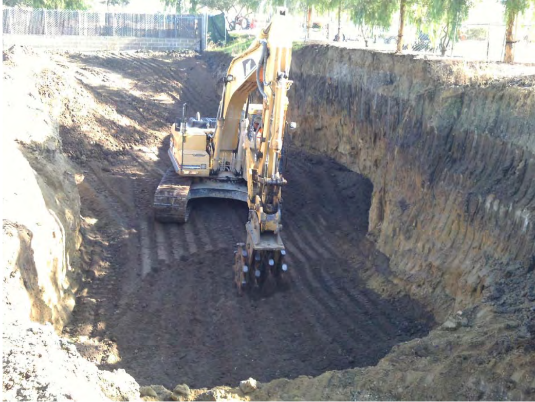
Photograph 3: Facing east during backfilling and compacting activities.
