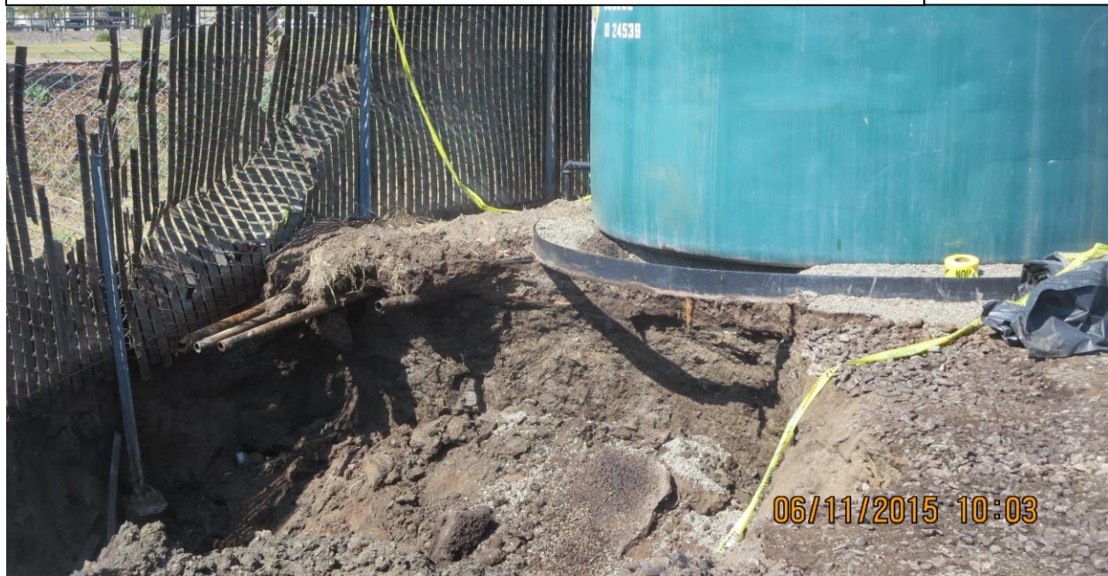
DESCRIPTION: SOUTHWEST VIEW OF EXCAVATION HOLE
