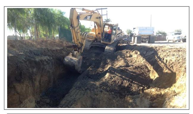
Description: Excavation of southwest stained soil in SW corner Photo # 1 of
