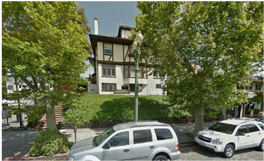
522 Grand Avenue (Looking North on Grand Ave.)
