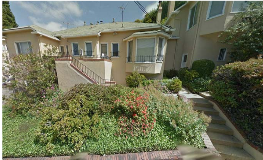
450 Euclid Ave. Part 2 (Looking North on Burk St.)
