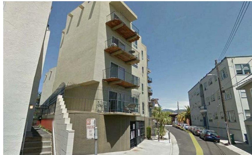
415 Lagunitas Ave. (Looking North East on Burk St.)
