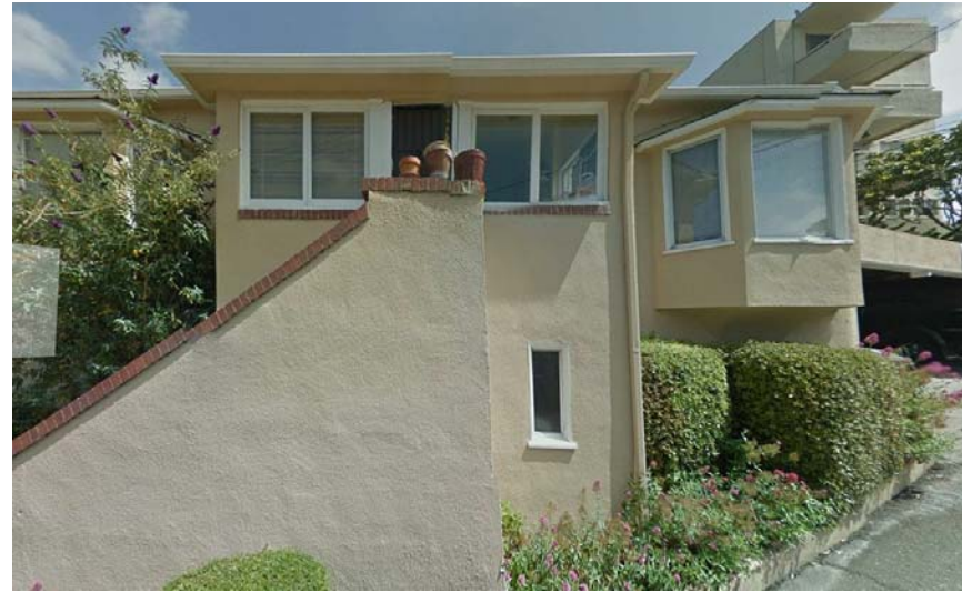
450 Euclid Ave. Part 1 (Looking North on Burk St.)
