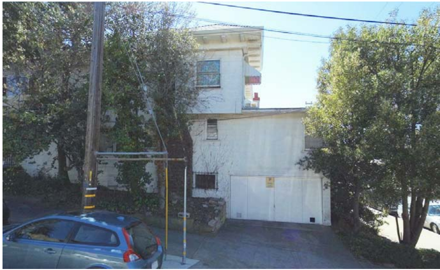
426 Euclid Ave. (Looking South on Lagunitas Ave.)
