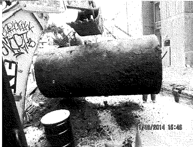
TANK REMOVAL IN PROCESS
