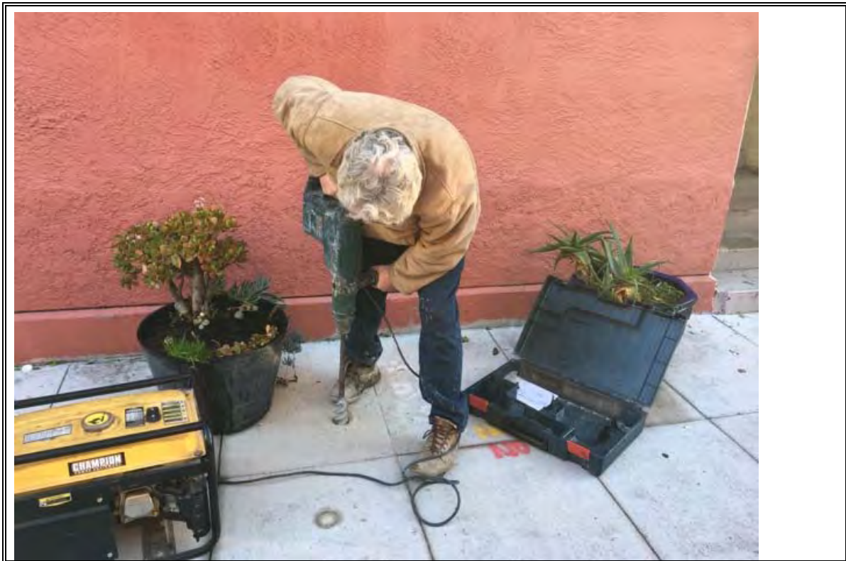
4. Sidewalk slab cutting for SV-2-5.
