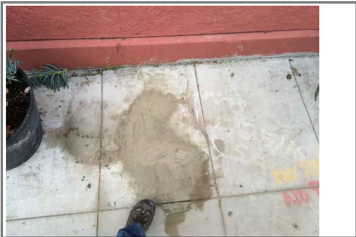
6. Sidewalk after grouting and patching.
