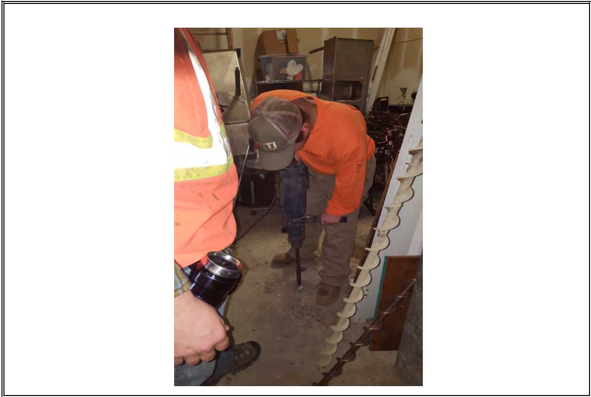
1. Concrete slab drilling for boring SV-1-3.
