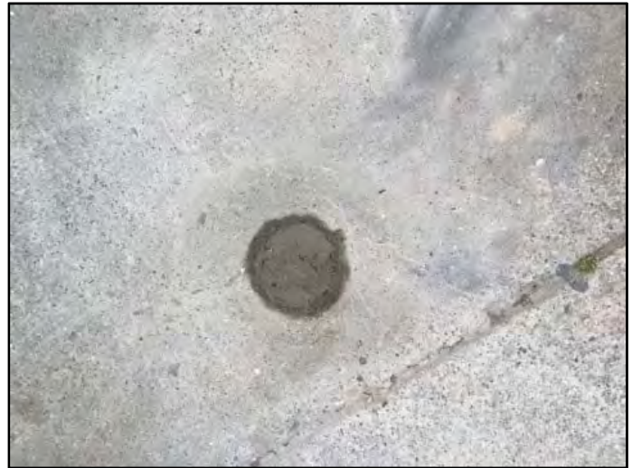
Photograph 4: The soil borings were backfilled to ground surface with Portland neat cement grout.
