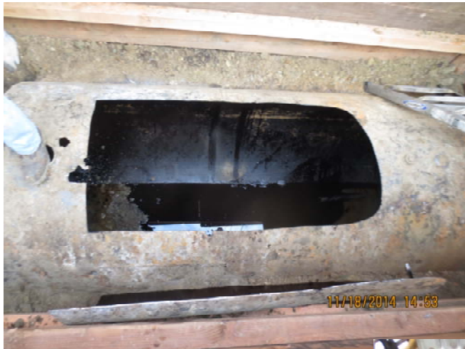
UST READY TO REMOVED FROM EXCAVATION
