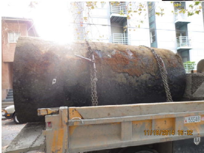
TANK READY TO BE TRANSPORTED FOR DISPOSAL
