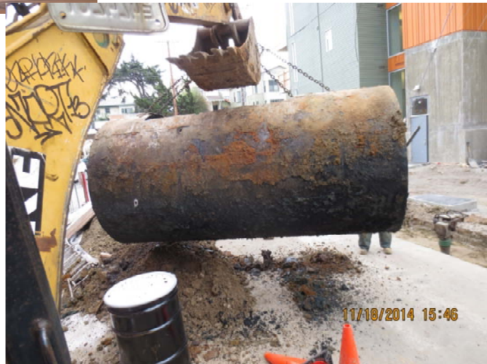
TANK REMOVAL IN PROCESS
