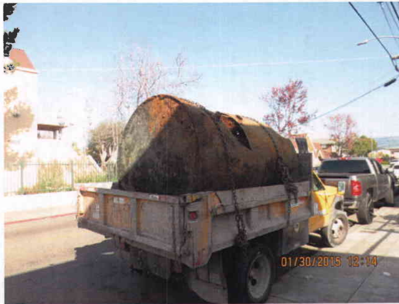
TANK SECTIONS READY TO BE TRANSPORTED FOR DISPOSAL
