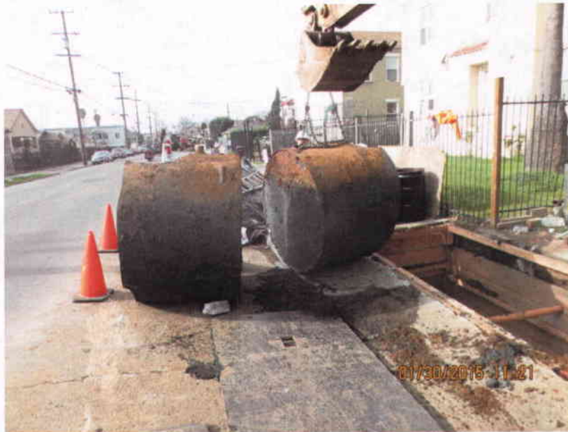
TANK REMOVAL IN PROCESS
