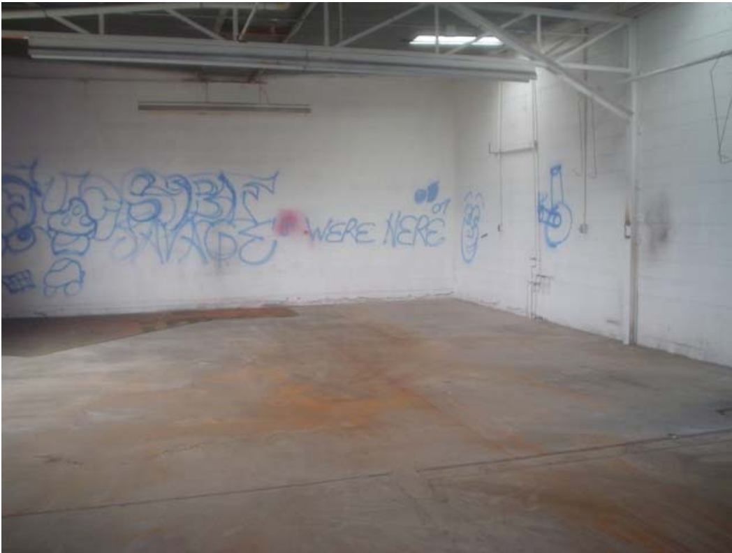
PHOTO #5. VIEW OF PORTION OF NORTHWEST END OF BUILDING.
