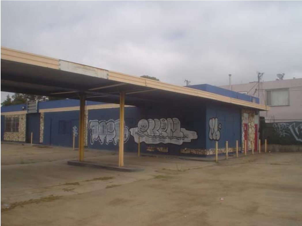
PHOTO #4. ADDITIONAL VIEW OF FORMER FUELING AREA.
