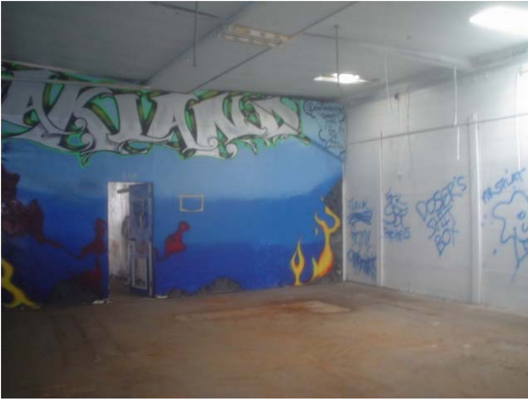
PHOTO #7. VIEW OF SOUTHEAST PORTION OF BUILDING.
