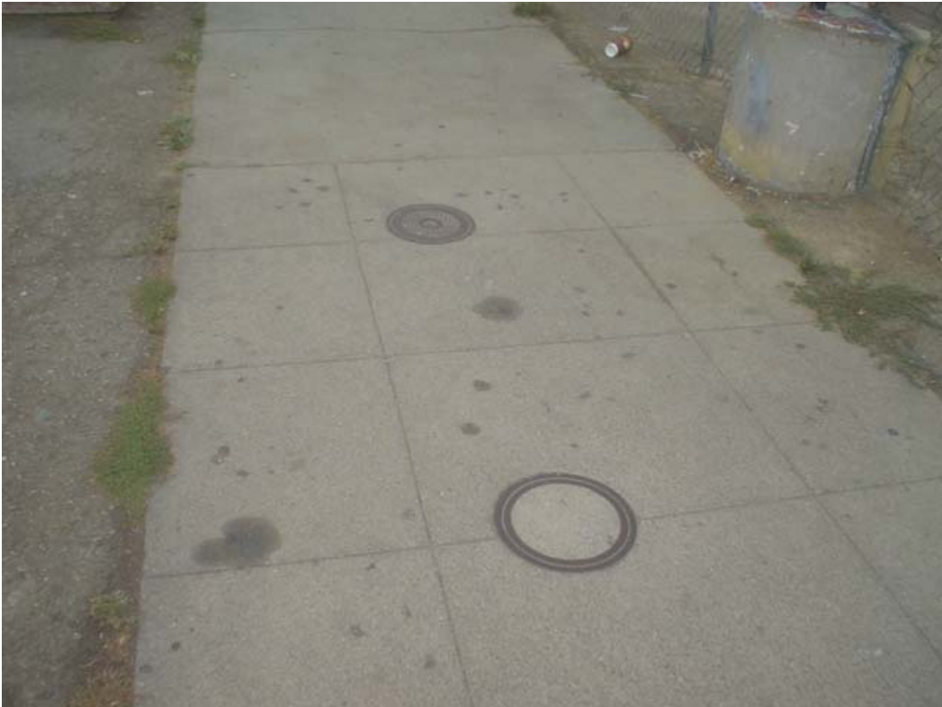
PHOTO #8. VIEW OF CHRISTY BOX AND SEALED BOX IN SIDEWALK.
