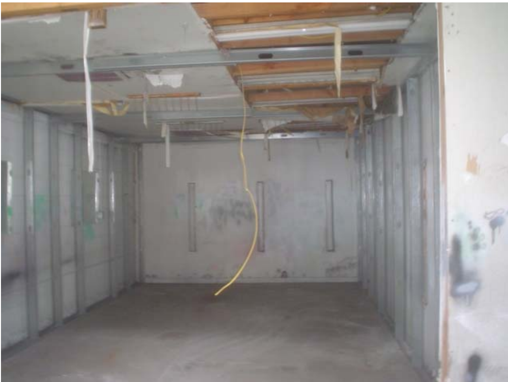
PHOTO #6. VIEW OF FORMER SPRAY BOOTH.
