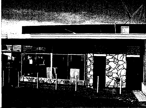
Photo #1: South side of Project, facing north
