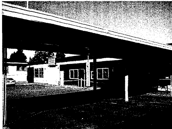
Photo #3: West side of Project, facing northeast
