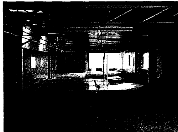
Photo #5: Interior of Project building
