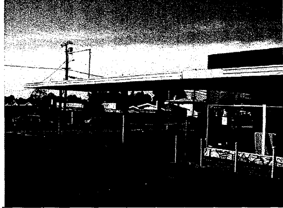
Photo #2: South side of Project, facing northwest
