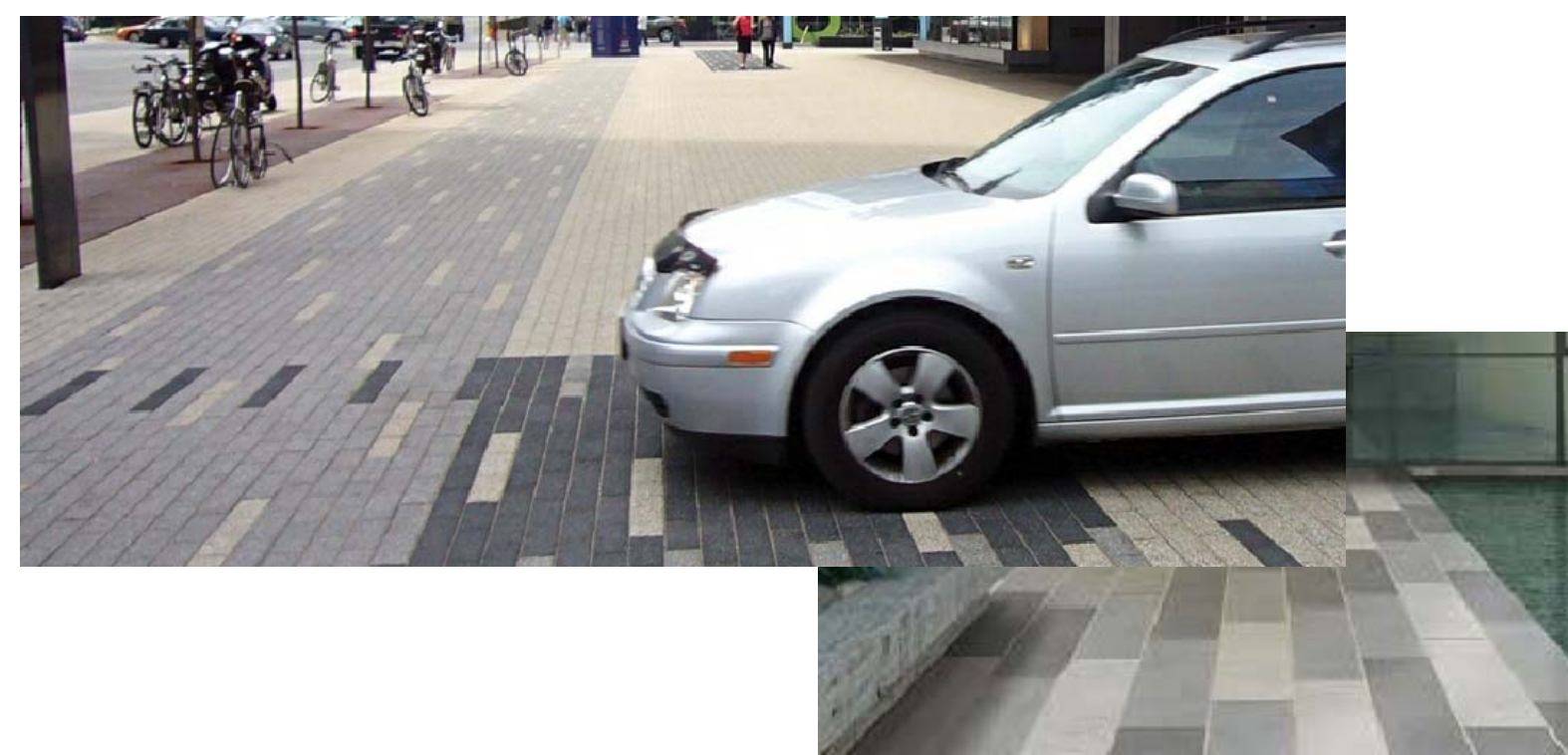
LARGE SCALE PERMEABLE VEHICULAR PAVERS IN DRIVE AISLE
