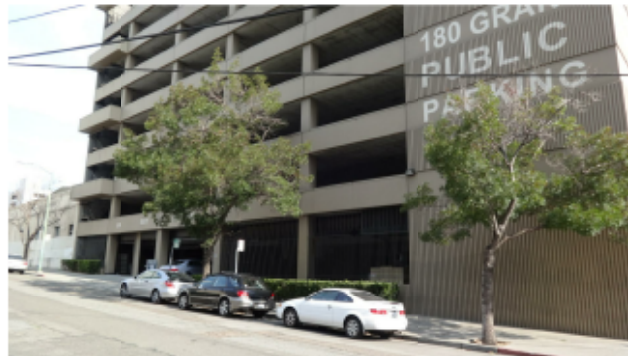
EXISTING 9-STORY PARKING GARAGE AT 23RD AND WAVERLY
