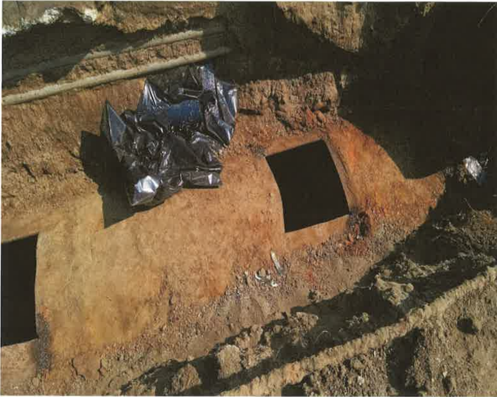
Photograph showing access holes cut into top of tank for cleaning
