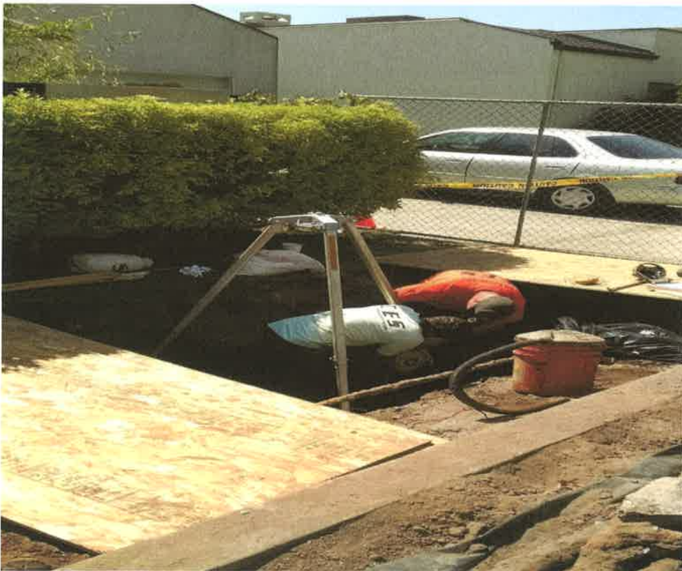
Tank cleaning operations
