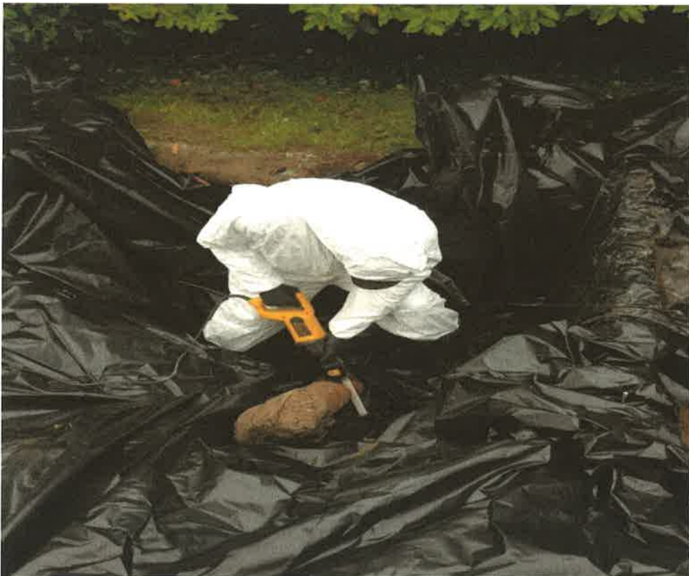
Photograph showing cutting of tank system piping
