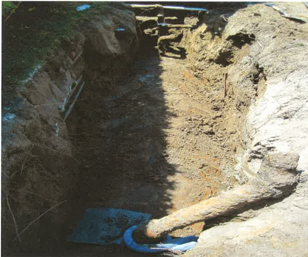
Surface of the tank showing both fill pipe and product delivery system manifold. The joint trench is visible to the left of the photograph
