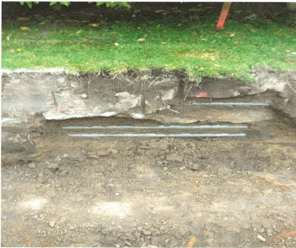
Photograph of joint trench located on south edge of tank excavation
