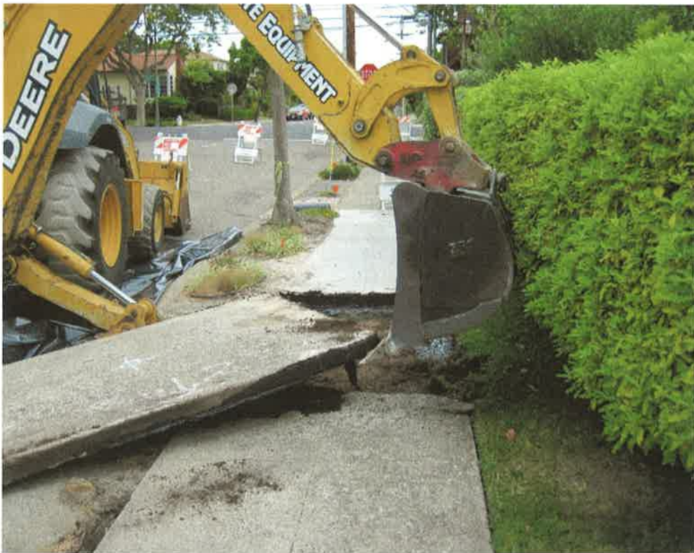
Additional photograph of sidewalk removal
