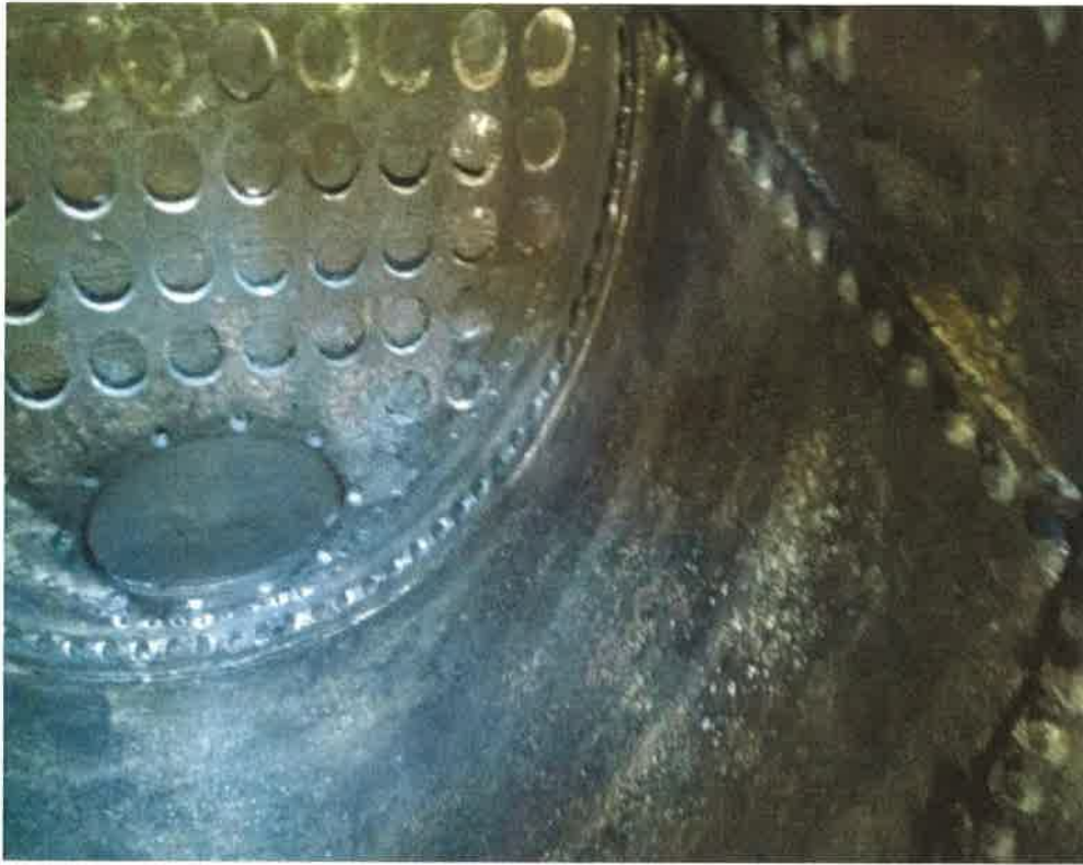
Inside surface of tank post cleaning
