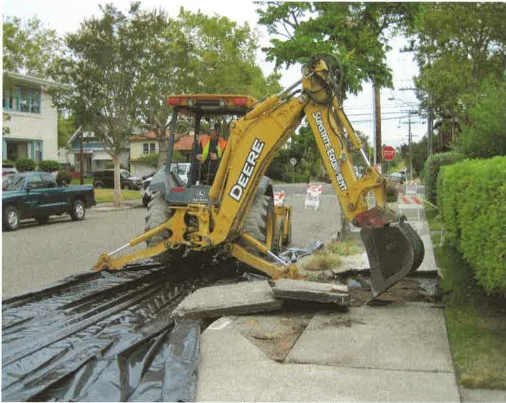
Photograph of sidewalk removal
