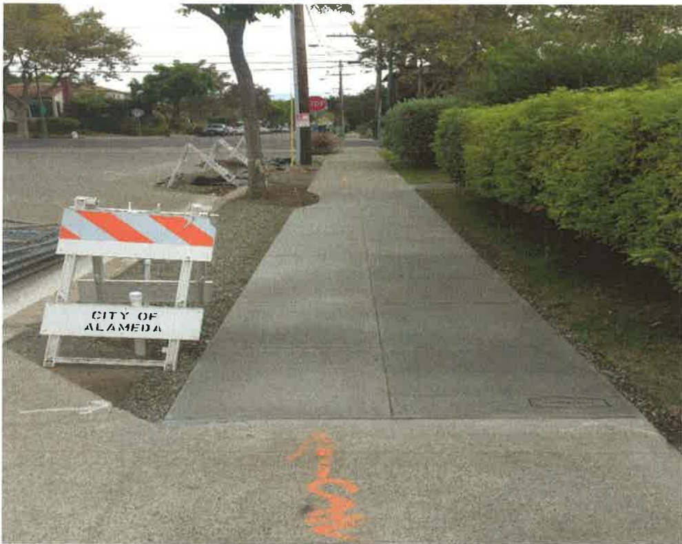
Restoration of sidewalk
