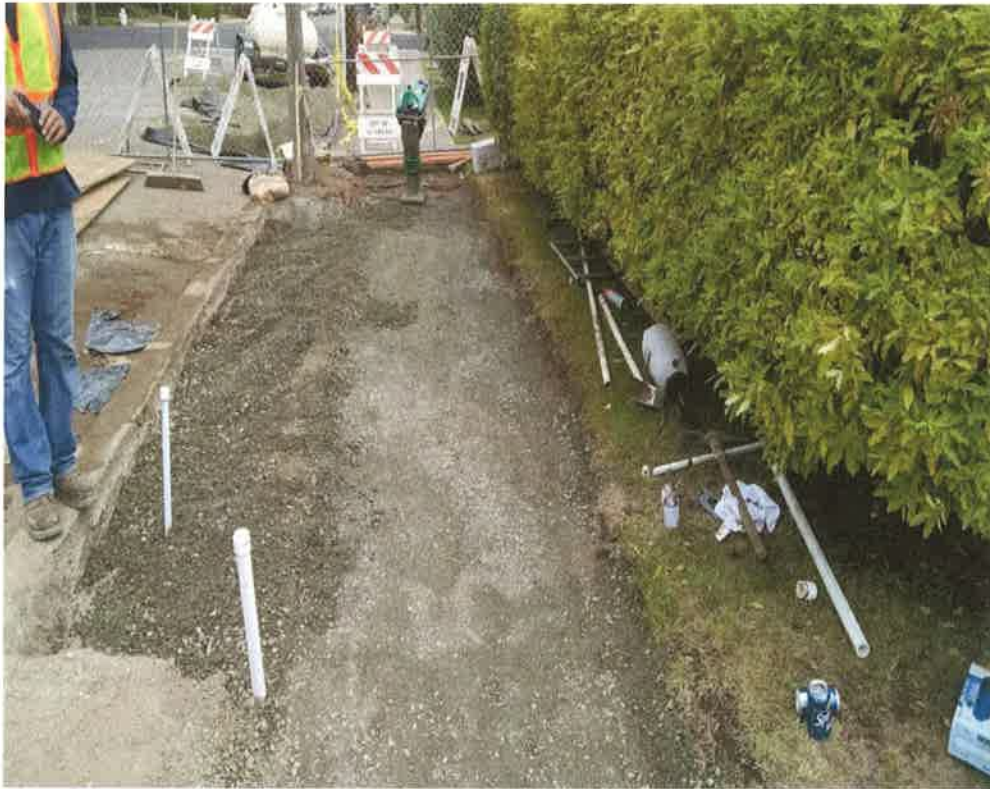
Backfill of excavation
