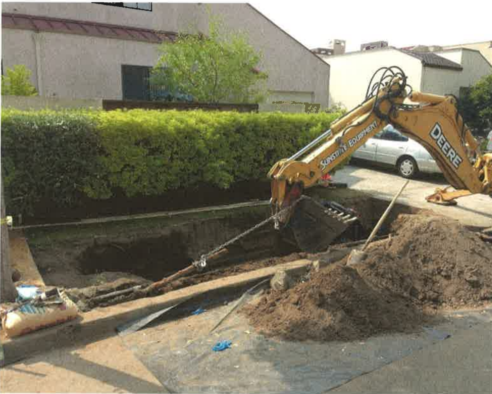
Removal of return line
