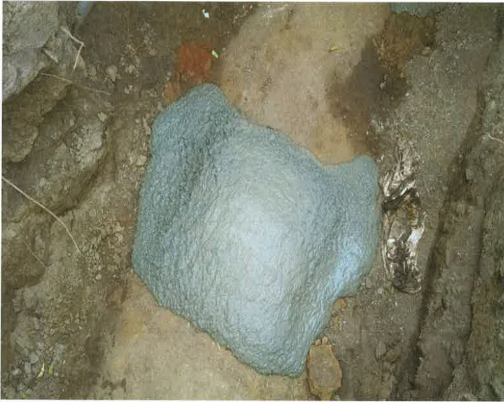
Overfill of CDF through access ports
