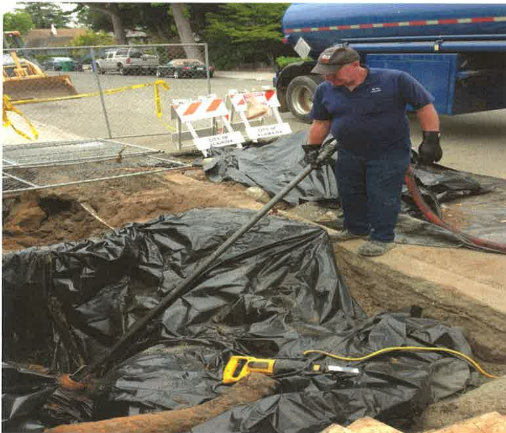
Product removal from tank
