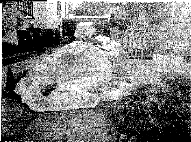
SOIL STOCKPILED ON VISQUEEN SHEETING
