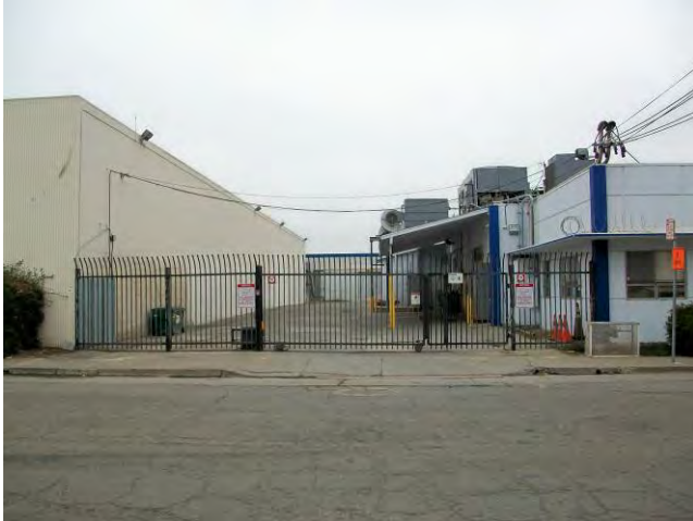
1. View northwest of gated entrance to subject property from Lesser Street.
