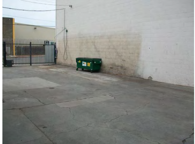
20. View south of solid waste bin staged in driveway near entrance gate.
