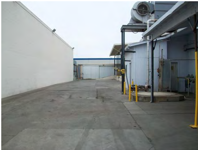
3. View northwest of interior driveway.
