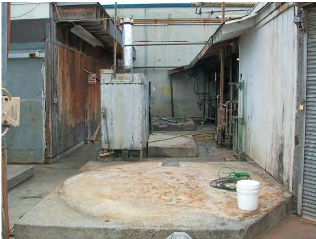
15. View of northeast of service area between Building 1 (at right) and Building 2 (at left).
