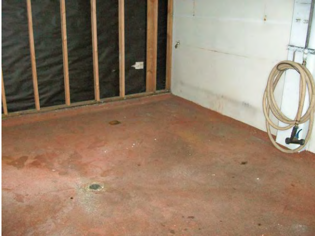
7. View of former food ingredients mix room in Building 1.
