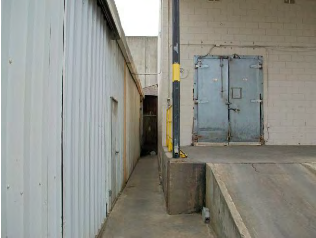
13. View northwest of Building 4 (dry storage building) southeast façade.
