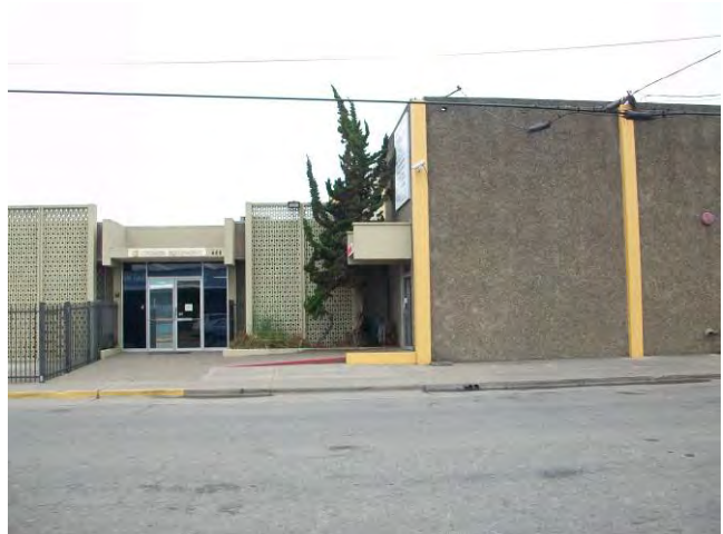
22. View of adjoining property to southeast across Lesser Street, Cromer Equipment Co.
