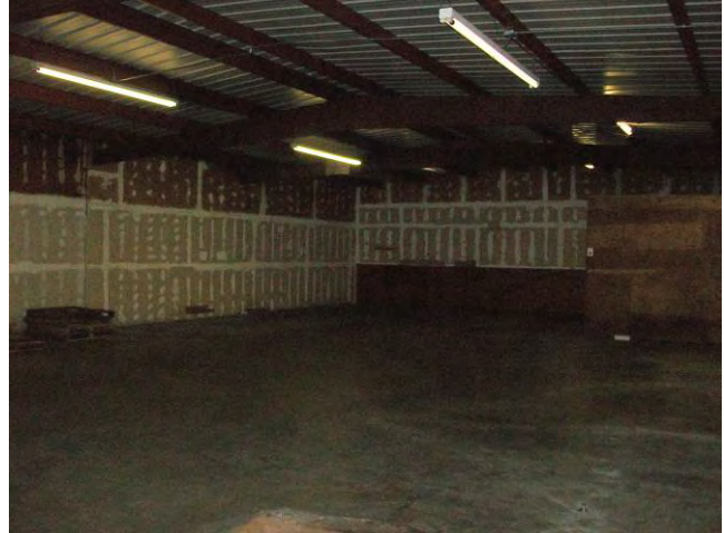
14. View Building 4 interior.
