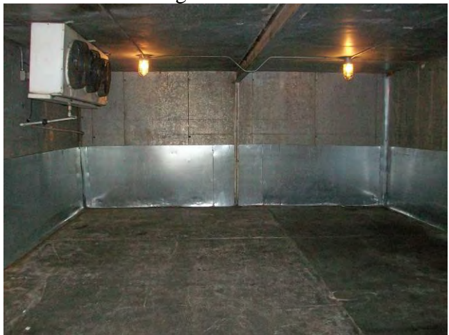
12. View of Building 3 freezer room interior (typical).
