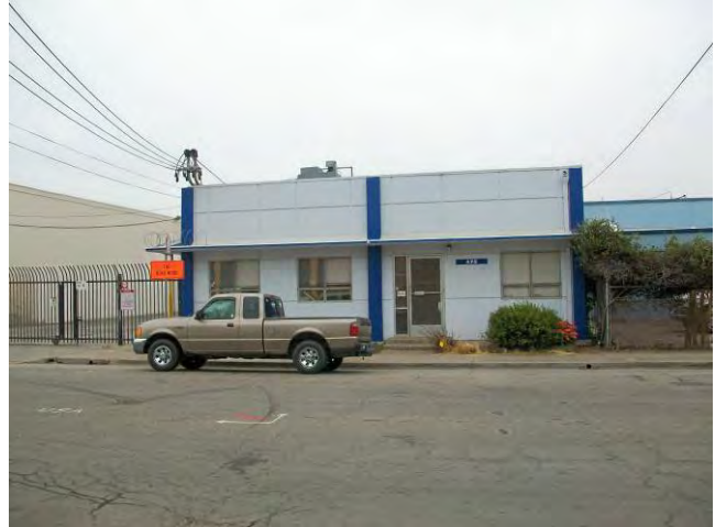
2. View northwest of Building 1 (office/former food processing building) southeast façade.
