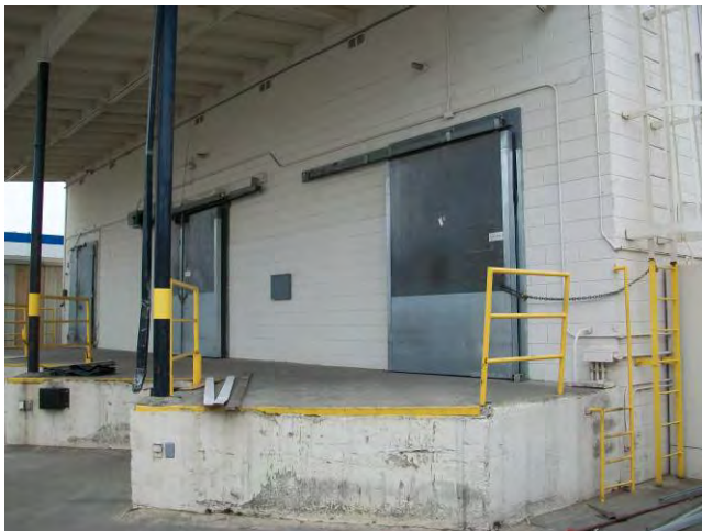
11. View north of Building 3 southwest façade and freezer rooms.
