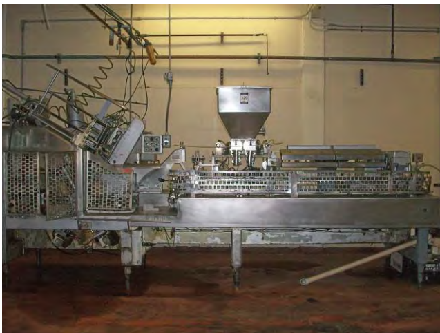
5. View of Building 1 idle food processing equipment.
