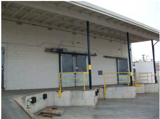
10. View east of Building 3 (cold storage building) southwest façade and refrigeration rooms.
