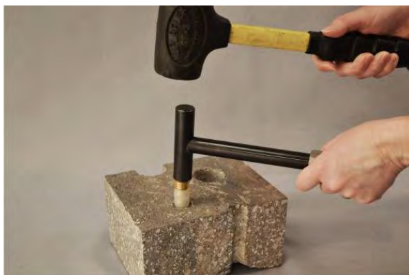
Figure 2. Installing the Vapor Pin™.
