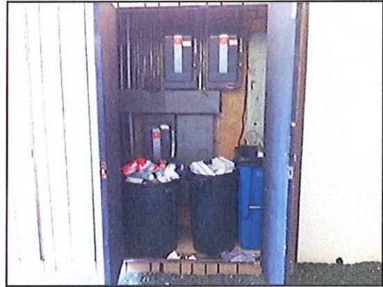
8 : Electrical/storage closet in entrance way of 1430 Franklin Street
