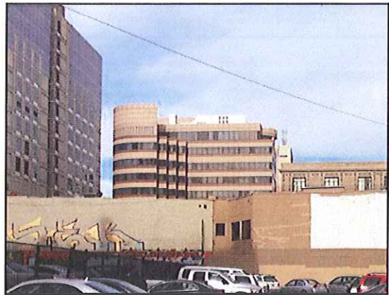
2 : Southeast side of the subject property as seen from the southwest
