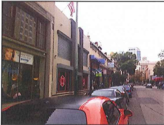
15 : Northeastern adjoining property as seen from 15th Street
