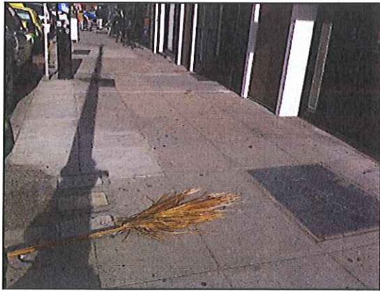
13 : Potential former location of heating oil underground storage tank
