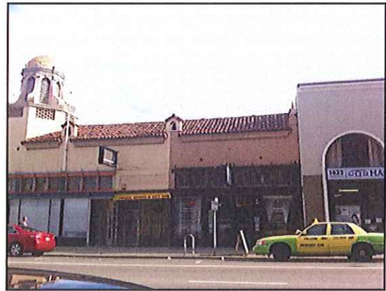
14 : Northeastern adjoining property as seen from Franklin Street
